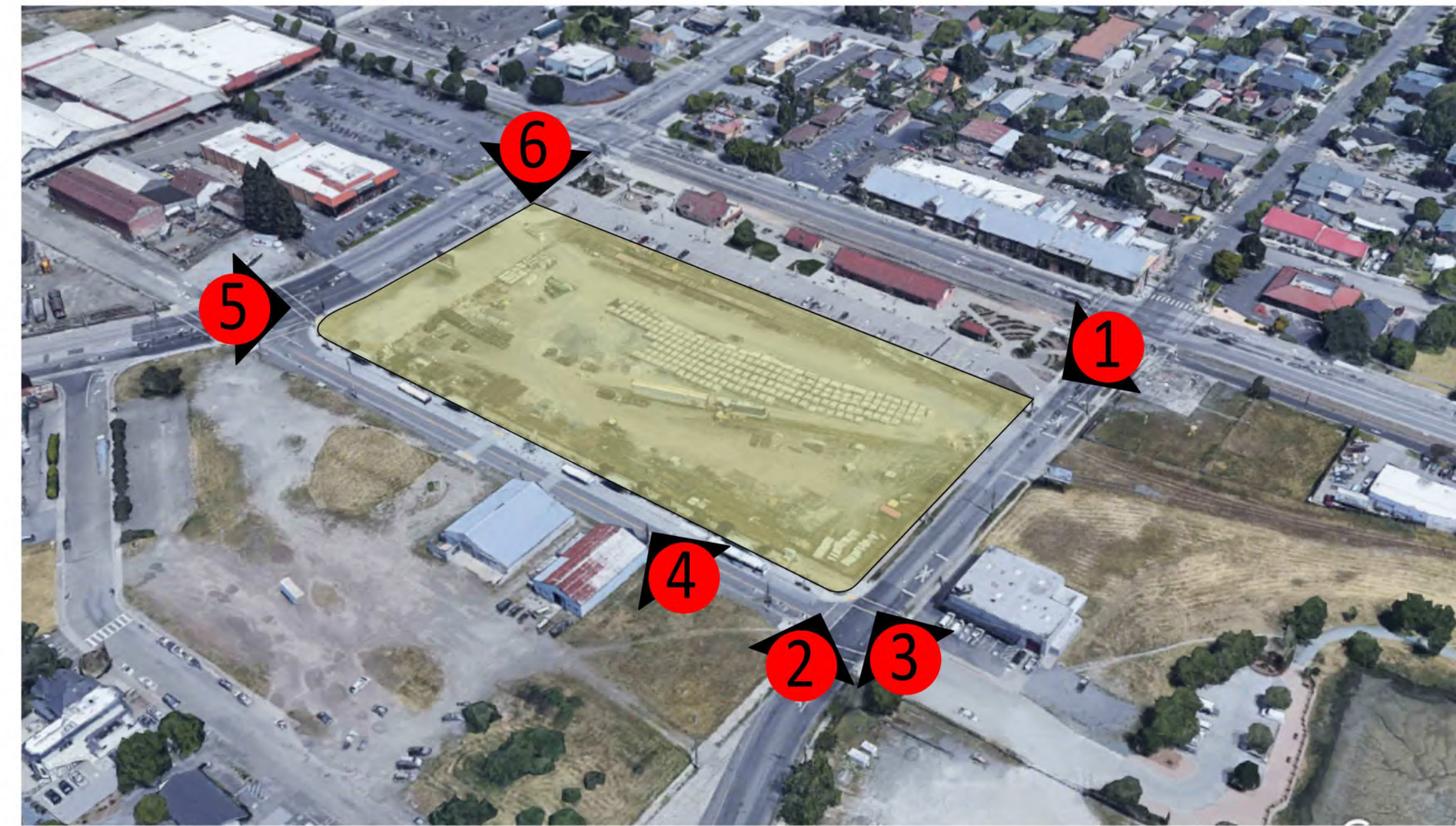
AERIAL VIEW OF SITE LOOKING NORTH
