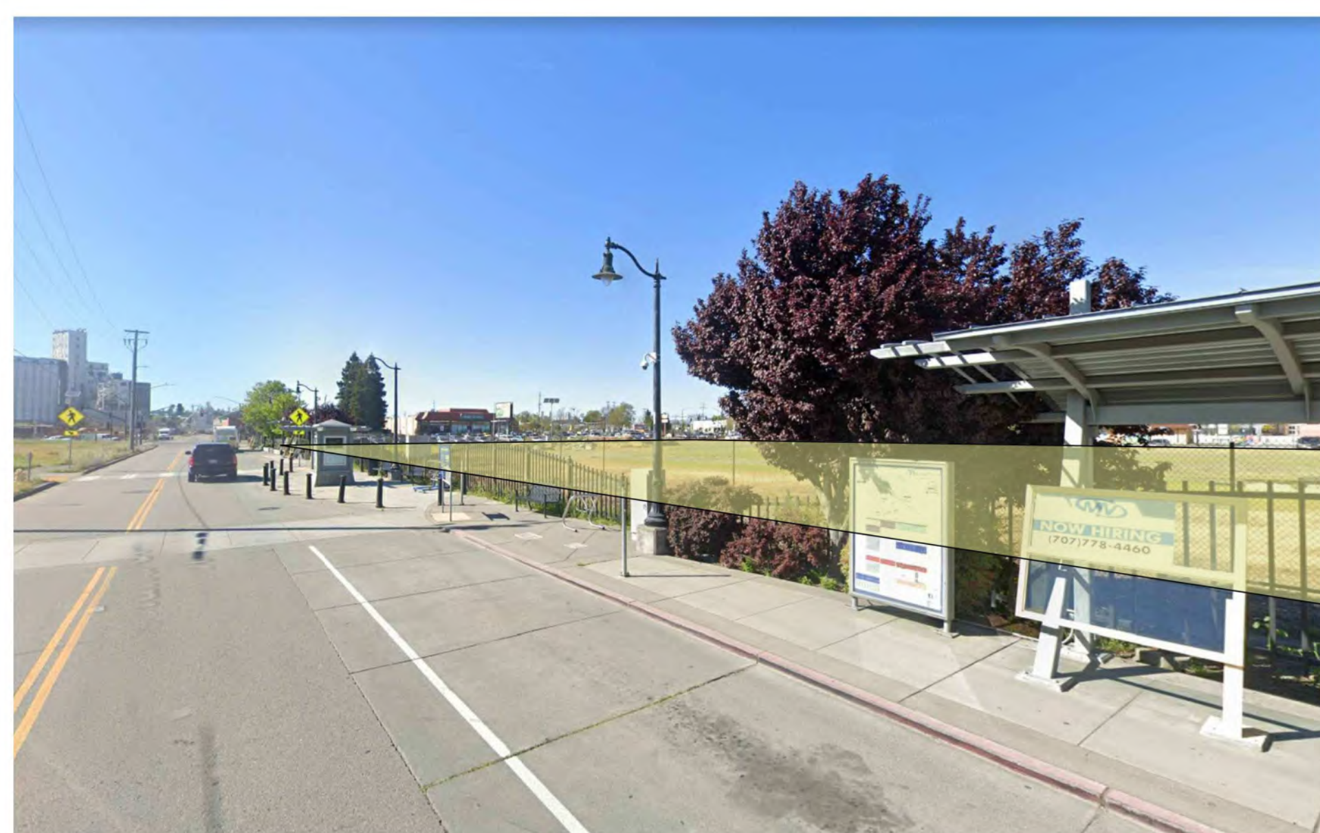
VIEW MID-BLOCK ON COPELAND LOOKING NORTH 4
