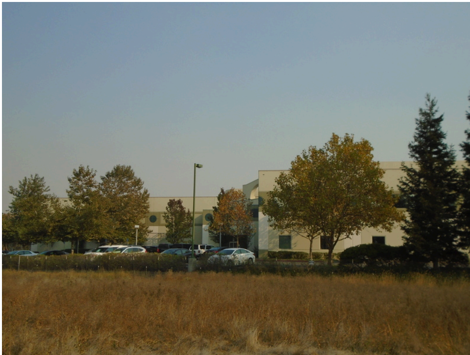
16. View of the northeast adjacent property from the west
