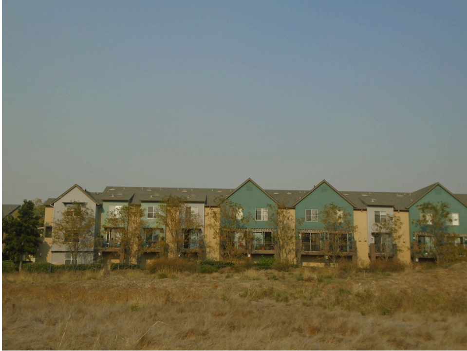
15. View of the north adjacent property from the south
