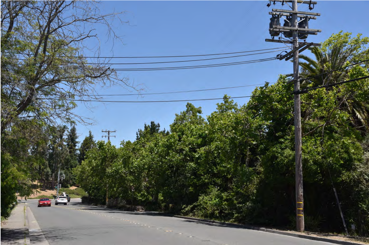
London plane trees are planted along Mc Near Avenue as street trees. All are subject to electrical line clearance pruning.
