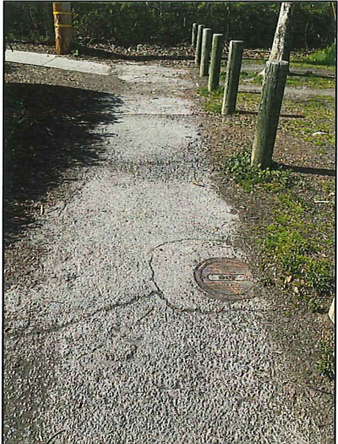
ADJUST VALVE BOX TO GRADE
