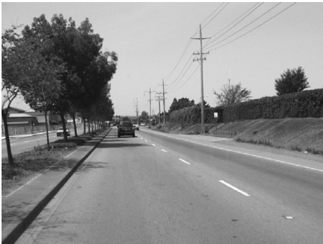
Lakeville Highway is a high speed corridor lacking in pedestrian amenities and scale; it represents a barrier between residential neighborhoods and access to nearby commercial and recreational opportunities.
