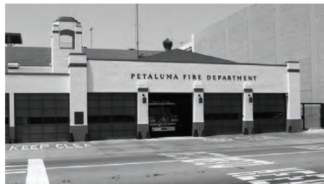
Fire Station 1 currently located on D Street will be replaced with a new facility on Petaluma Boulevard South.
