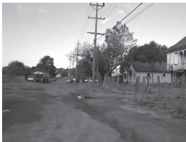
Unfinished street cross-sections, such as this segment of Shasta Avenue shown above, create opportunities to implement new street types at such time as these streets are fully improved with curb, gutter, landscape strips and sidewalks.
