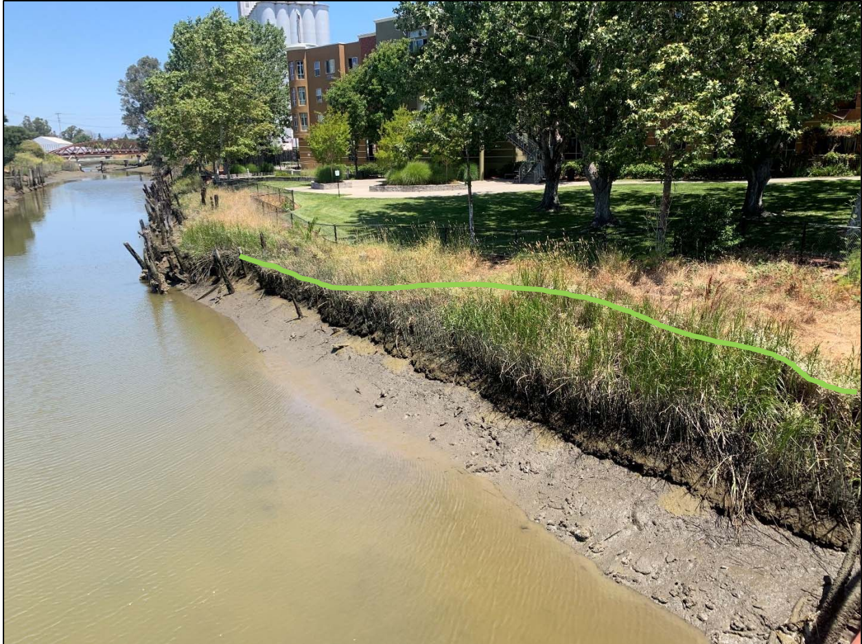
Photo 1. Approximate Location of High Tide Line (Green) along Eastern Bank of Petaluma River
