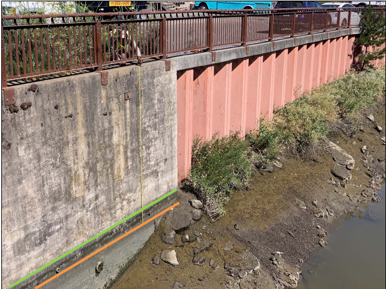
Photo 2. Location of High Tide Line (Green) and Mean High Water (Orange) along Western Bank of Petaluma River
