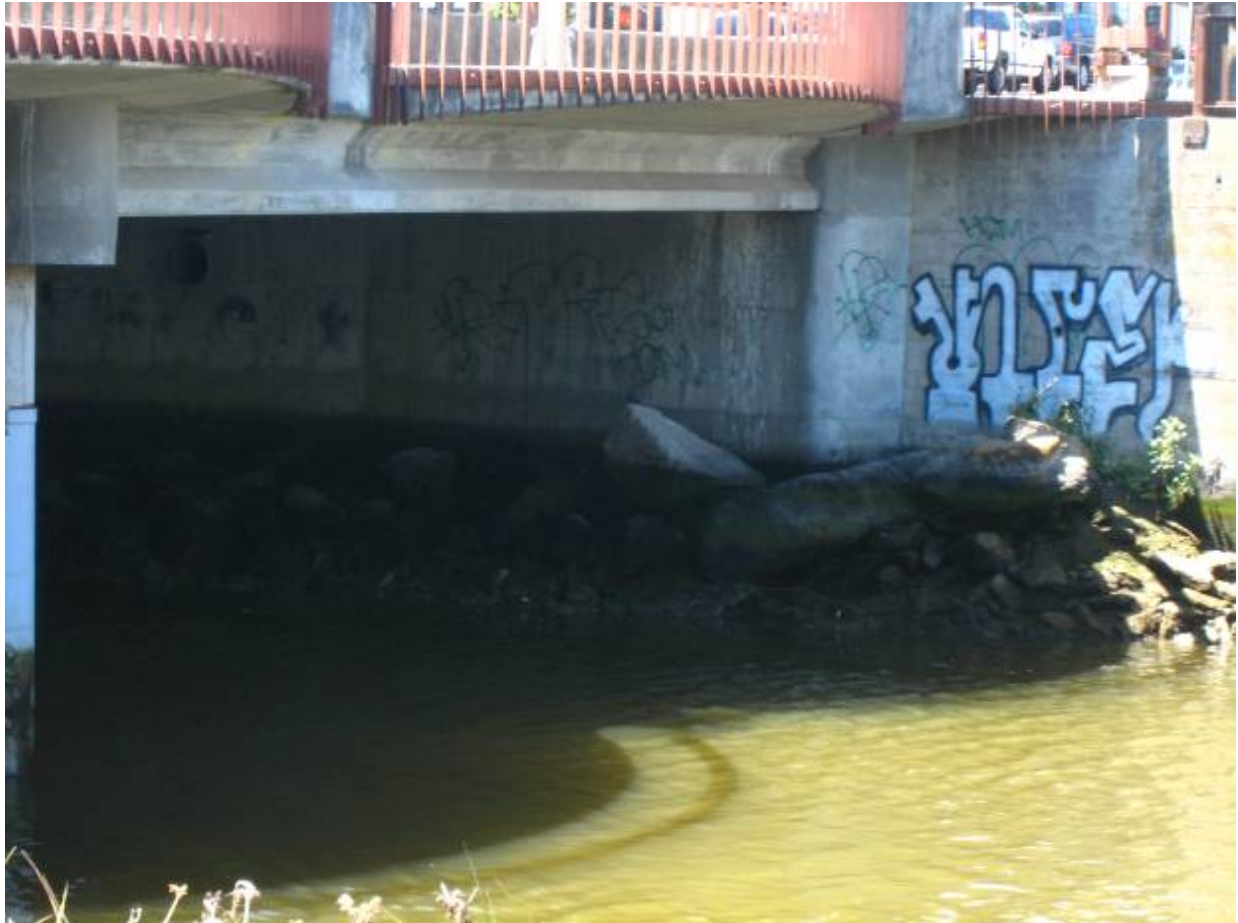
Abutment 1 – north side
