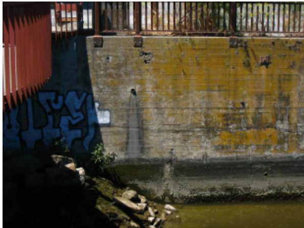
Retaining wall – north side
