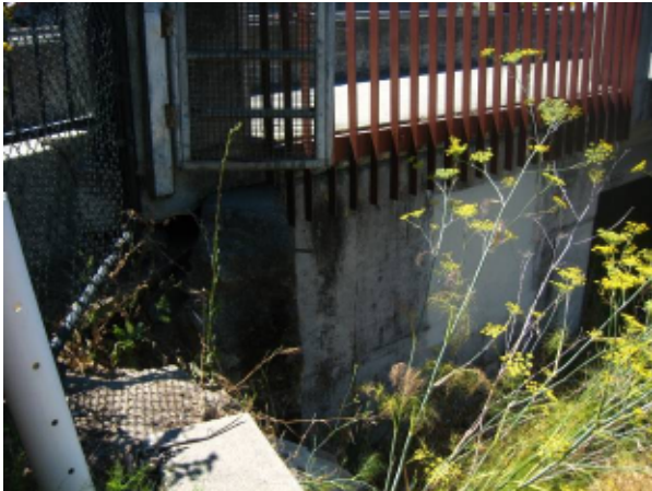
Remains of old abutment at wingwall
