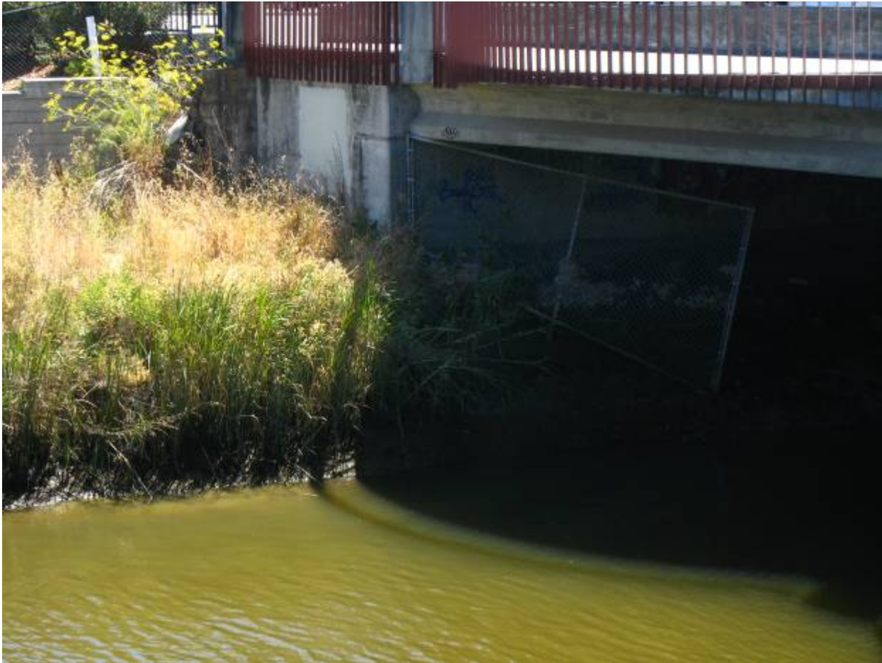
Abutment 3 – north side
