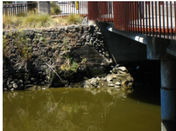
Retaining wall – south side
