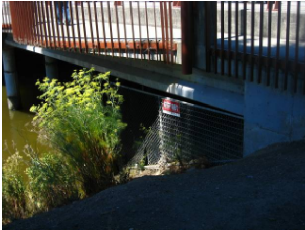
Fence under bridge
