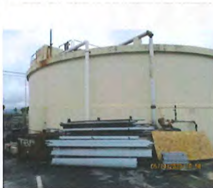
Showing the Primary Digester with existing coatings.
