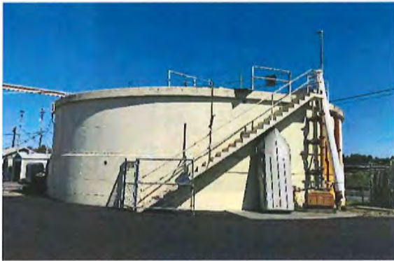
Figures 13 and 14. Primary digester (left) and secondary digester (right).
