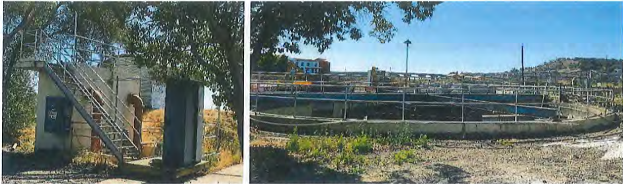
Figures 19 and 20. Secondary sludge structure (left) and secondary clarifier (right).
