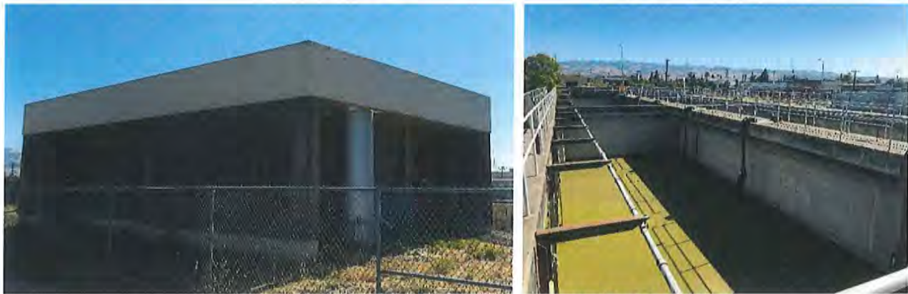
Figures 21 and 22. Blower building (left) and aeration tanks (right).
