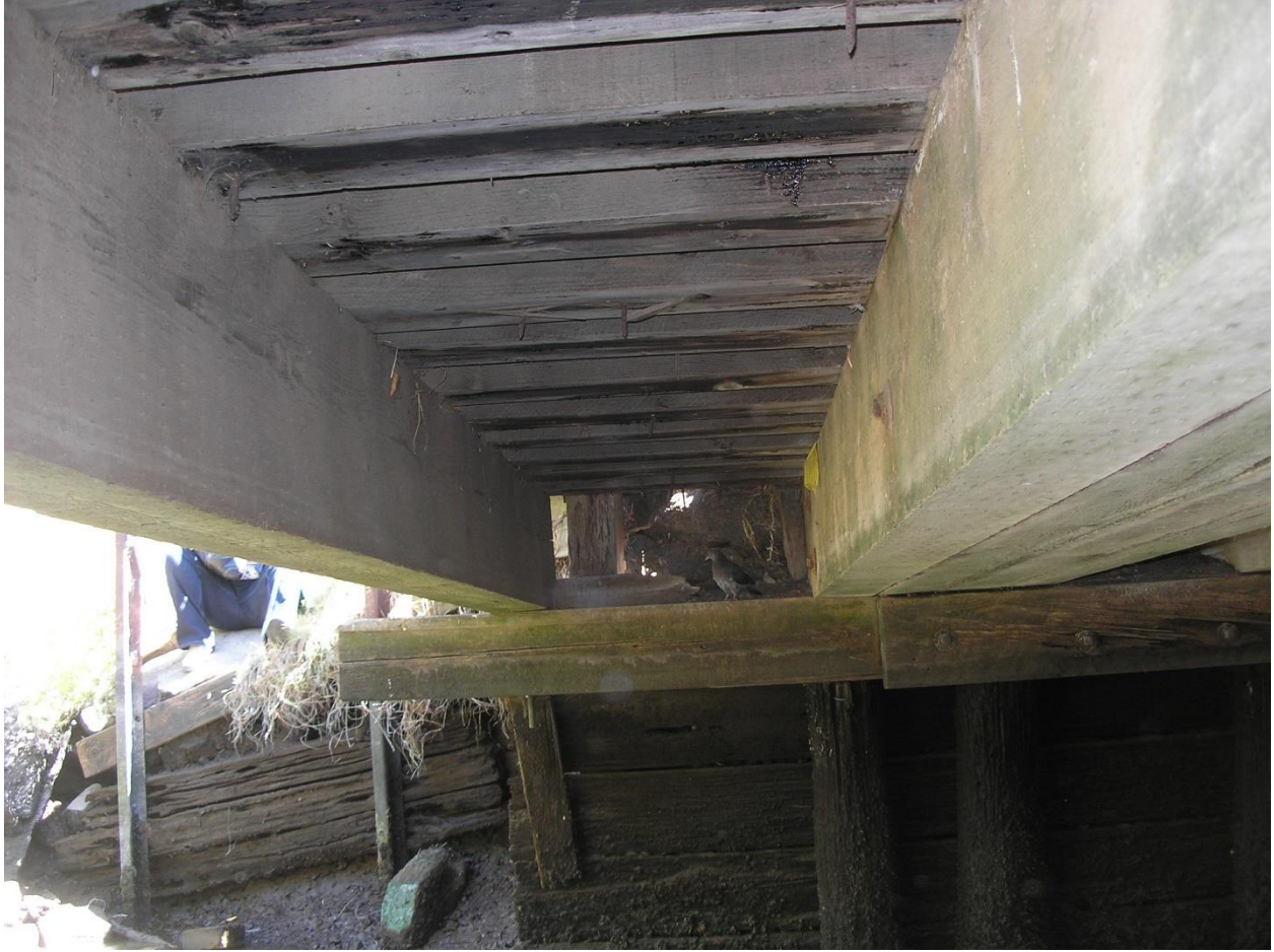
Below Deck 3 – 1 st and F St.
