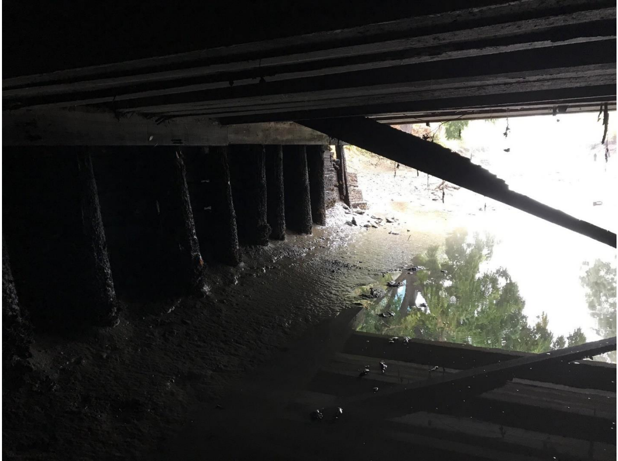
Below Deck 2 – 1 st and F St.
