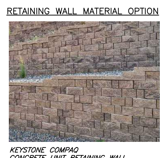
KEYSTONE COMPACT CONCRETE UNIT RETAINING WALL
