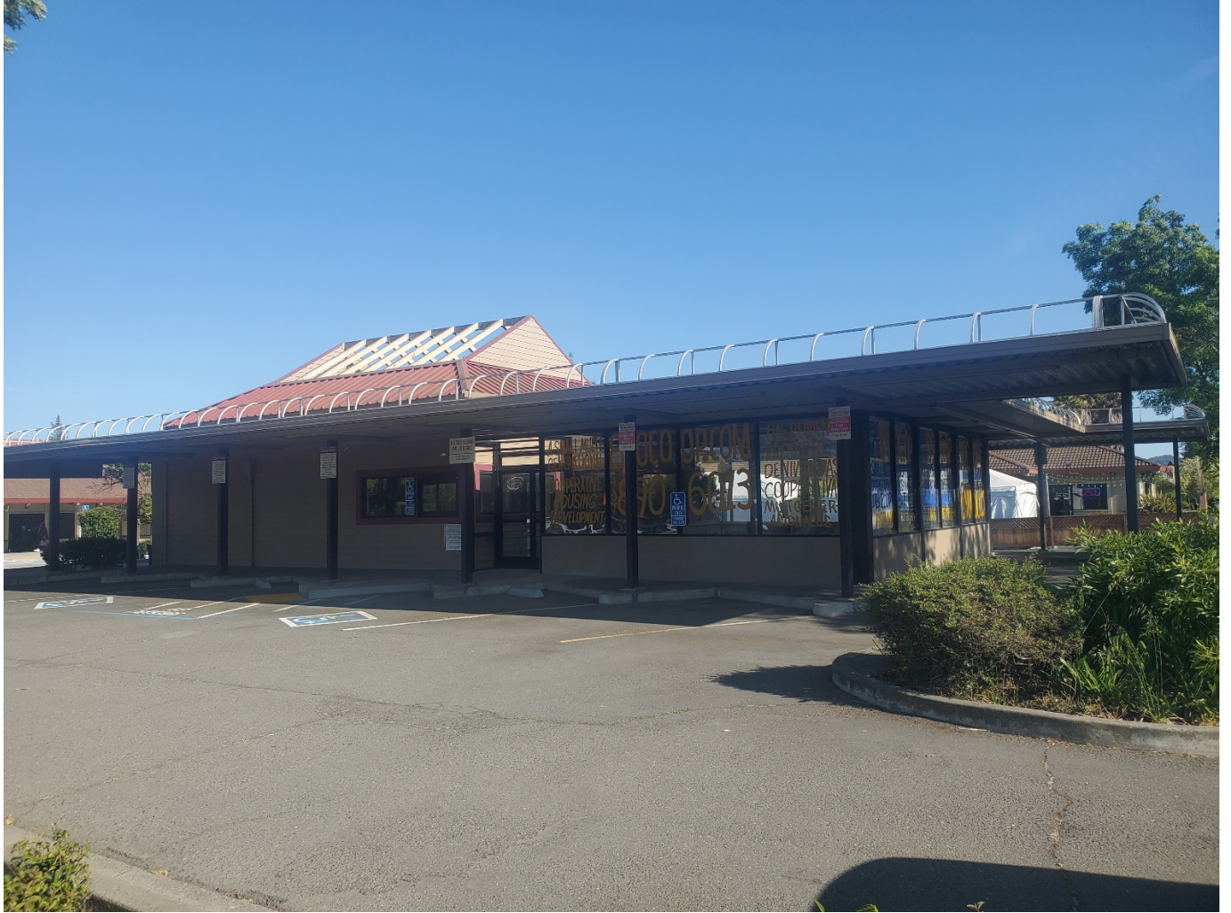
Existing Structure Viewed Looking Southeast
