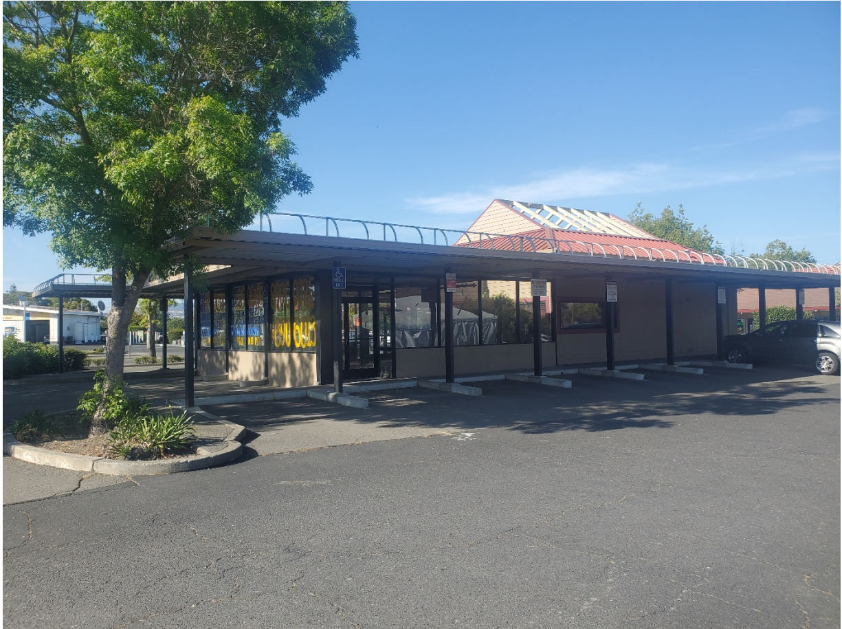
Existing Structure Viewed Looking Northeast
