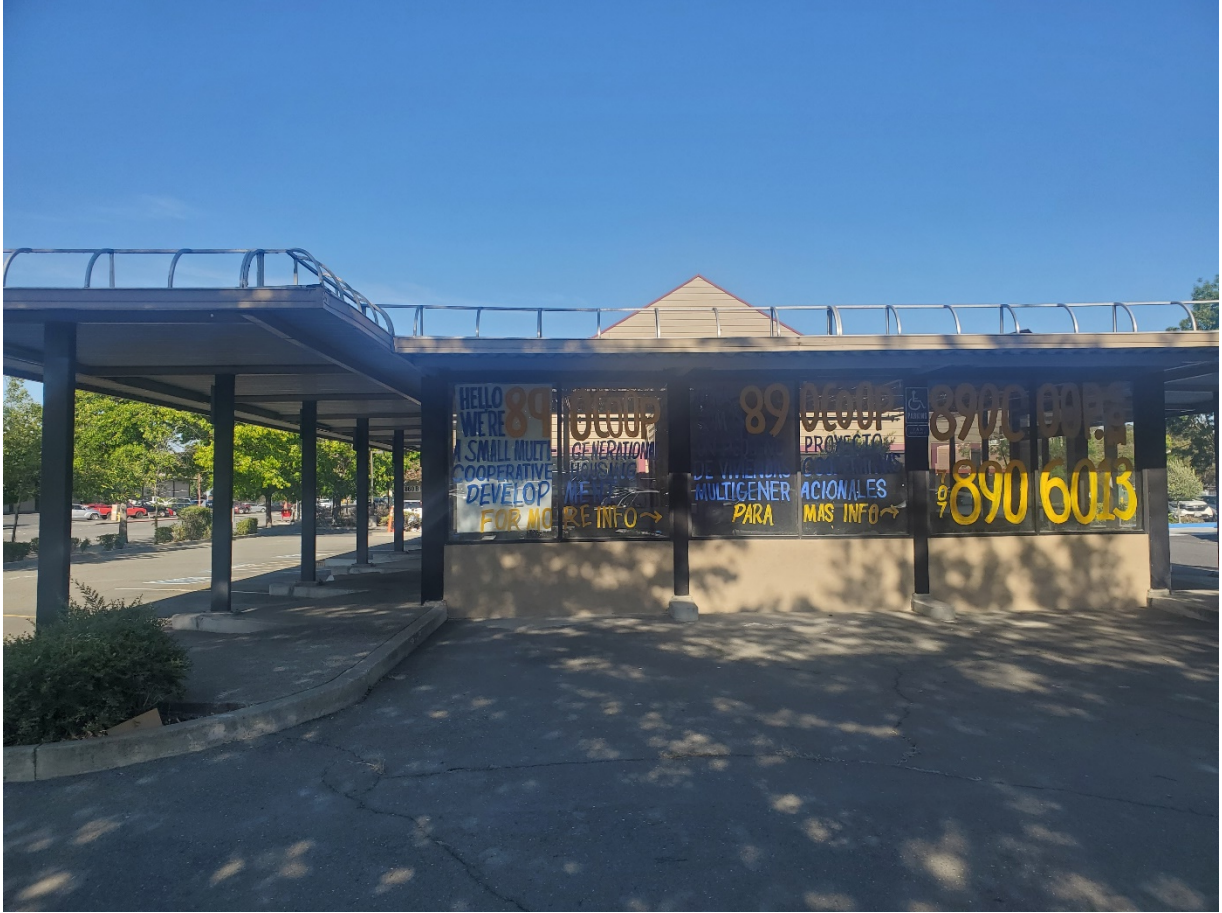
Existing Structure Viewed Looking East
