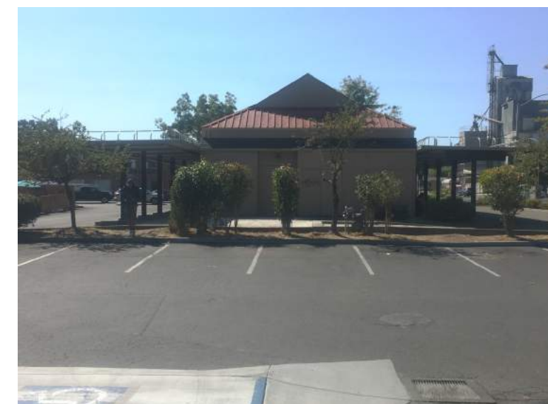
8 View of east side of building (rear side)
