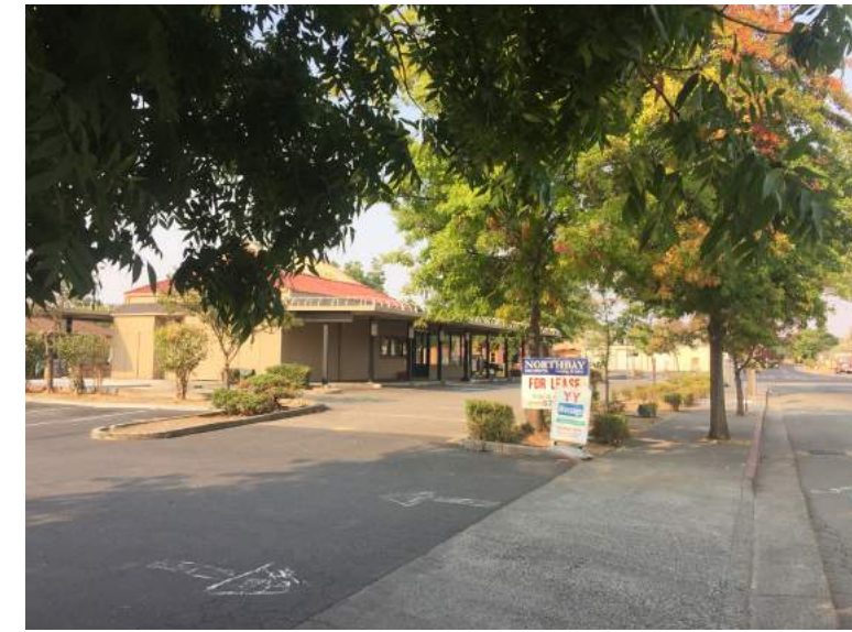
2 View of West Payran Street frontage
