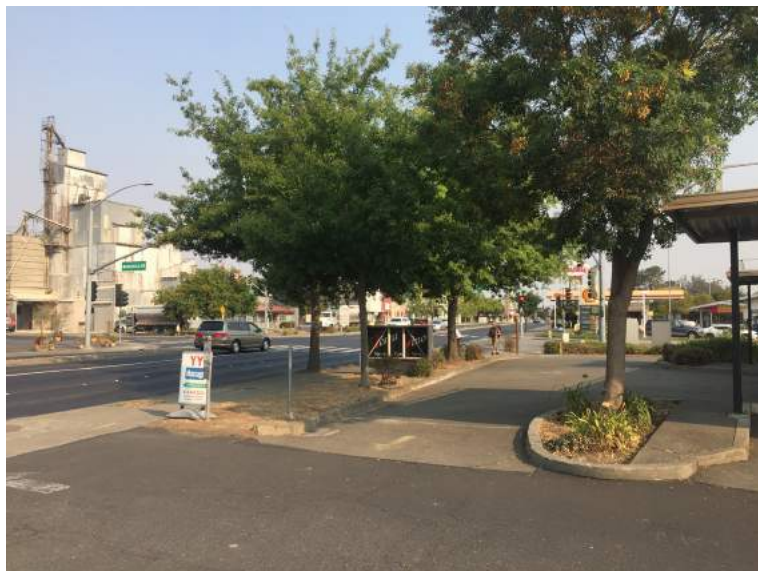
6 View of Petaluma Blvd N frontage from south drive aisle
