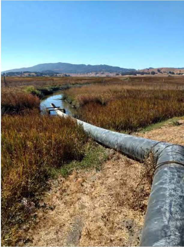
Photo 1: View of existing emergency outfall and pipeline located in slough. Replacement outfall will be similarly located, upland portion of pipeline will be buried.
