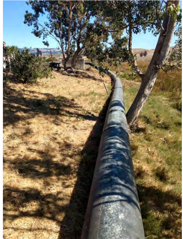
Photo 2: View of existing emergency outfall pipeline in uplands, looking west.
