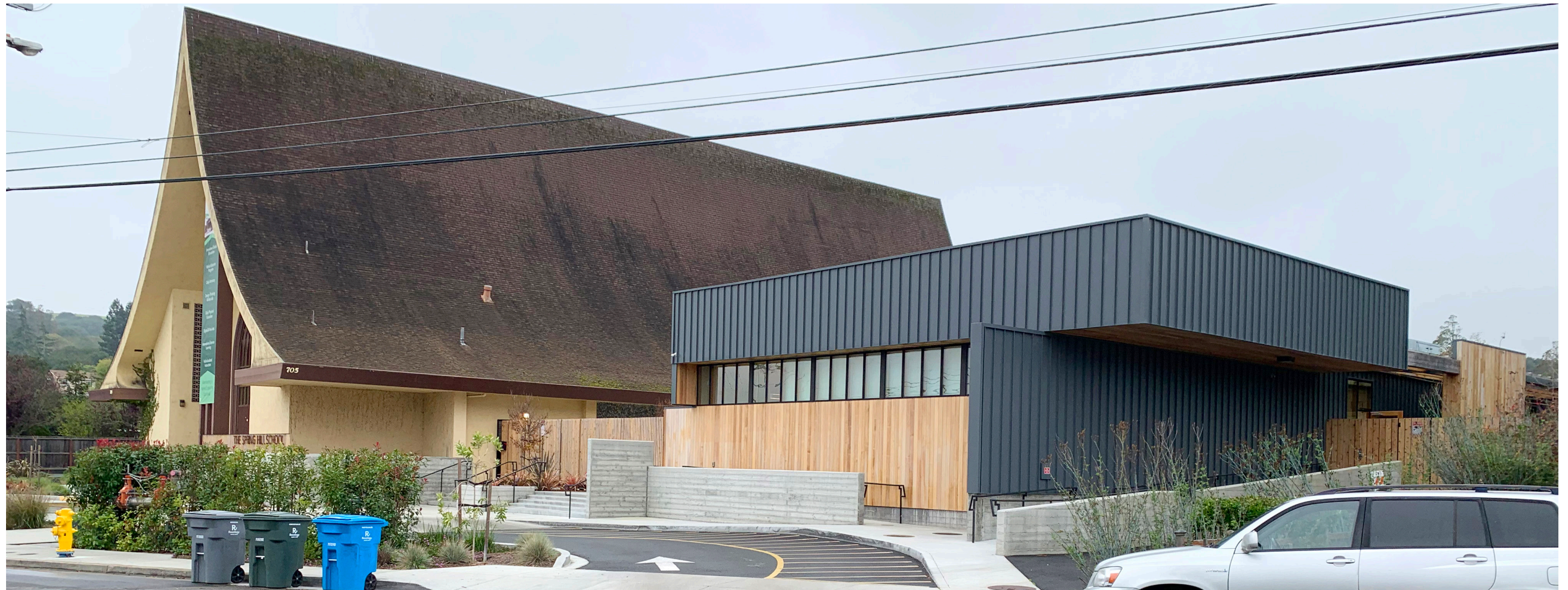
STREET VIEW OF EXISTING SCHOOL
