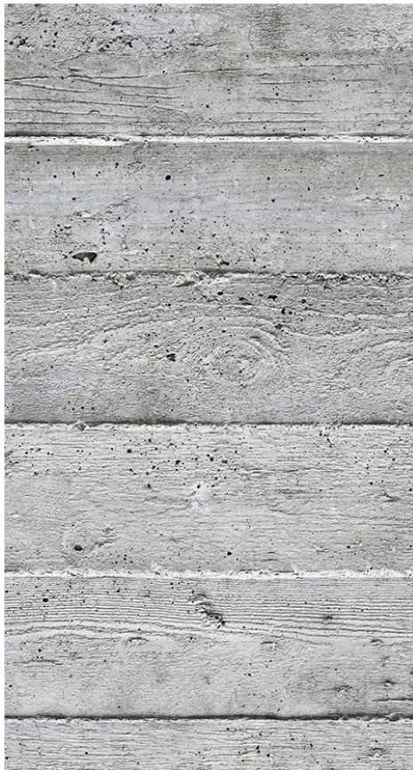
BOARD FORM CONCRETE
