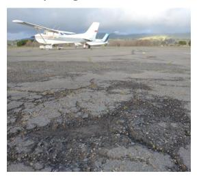
heavy rains accelerate the pavement's deterioration and necessitate rehabilitation. The Federal Aviation Administration (FAA) has already paid for the design. The construction of this project is reimbursable from the FAA and Caltrans Division of Aeronautics.
