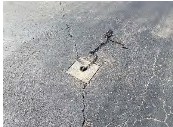
Photo 6: Existing Tie-Down Anchor
