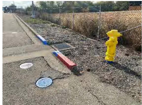
Photo 4: Existing Water and Drainage Features
