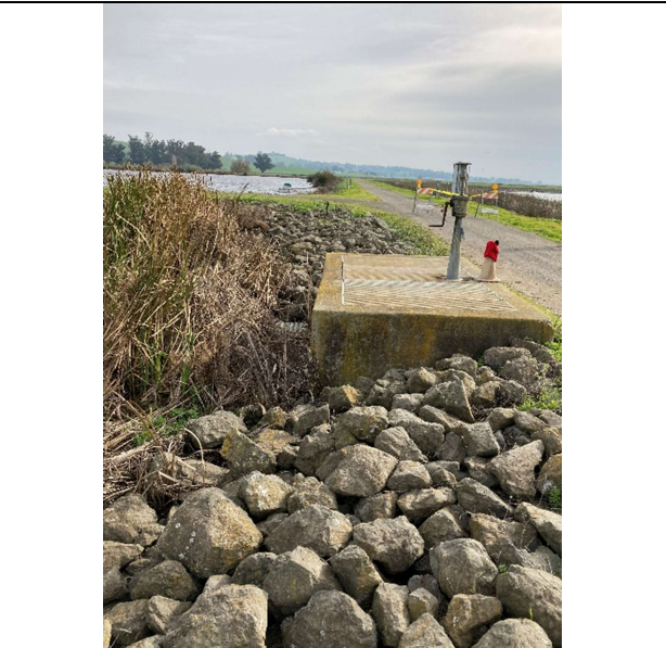
Aerated Lagoon to Pond No. 4 transfer structure.
