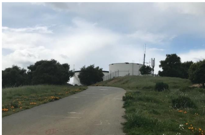
Figure 1: La Cresta tank site
