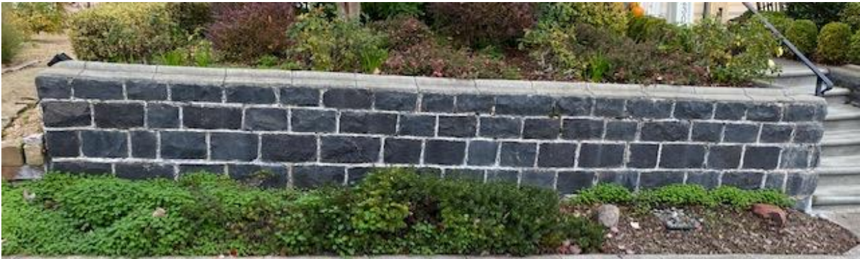
Basalt Retaining Wall at 230 Liberty St
