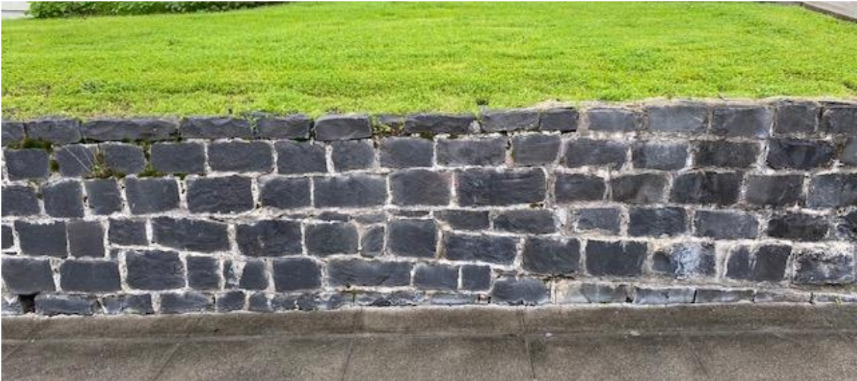
Basalt Retaining Wall at 231 Liberty St
