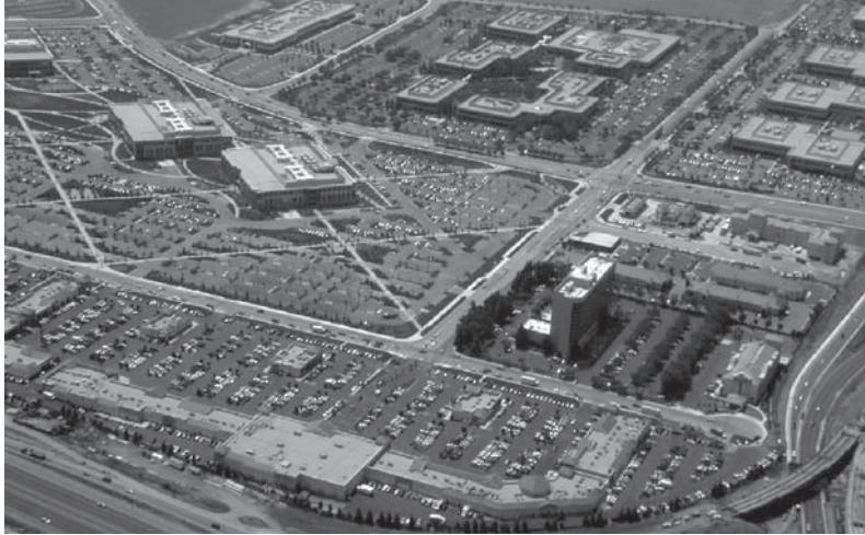
Figure I-1 Office park in San Jose
