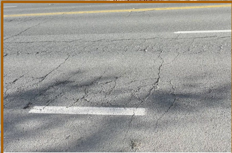
The pavement is in poor condition
