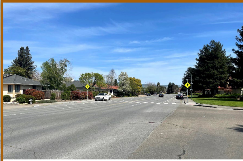
Long & uncontrolled crossings
