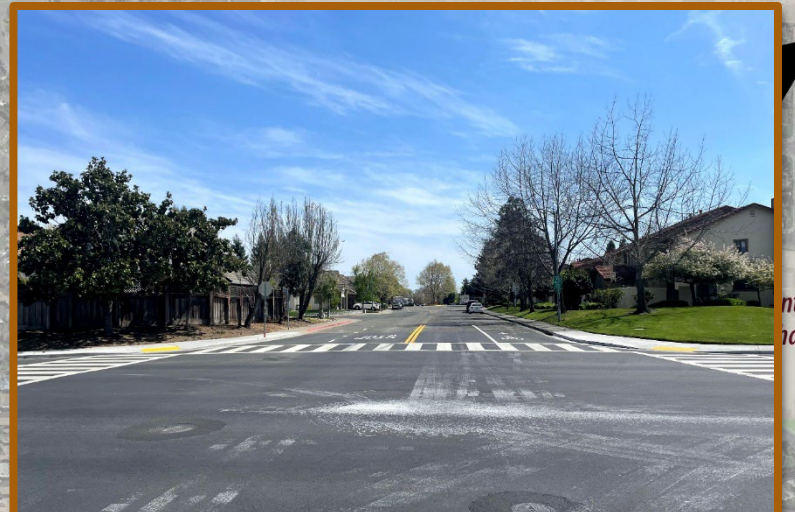
Recent upgrades on Maria Drive
