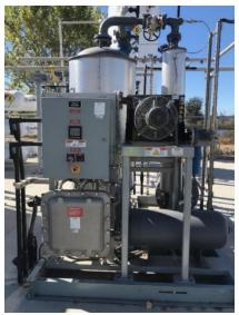
The anaerobic digester at ECWRF produces methane gas used to fuel a boiler to heat sludge. The excess methane gas is flared off. With the construction of another digester and the addition of high-strength waste to the treatment process, the plant will produce nearly double the amount of methane gas. The gas will be scrubbed, compressed, and used to fuel both City and Recology vehicles.
