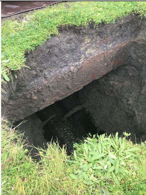
Exposed concrete for electrical line.
