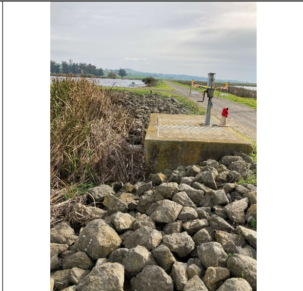
Aerated Lagoon to Pond No. 4 transfer structure.
