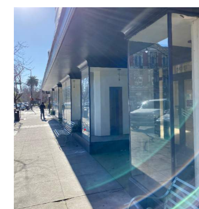
(E) STOREFRONT AND AWNING AT ENTRANCE
