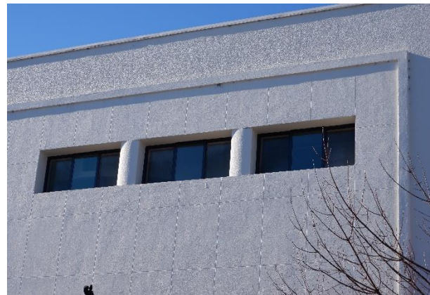
Figure 6. Three horizontally oriented windows on the east façade.
