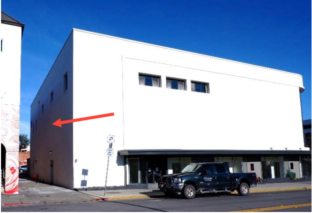
Figure 7. West façade (left) facing Telephone Alley indicated by red arrow.
