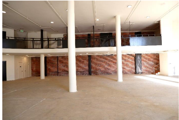
Figure 10. Mezzanine along the north wall.
