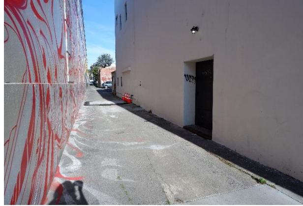
Figure 8. Pedestrian door at the west façade, looking north.
