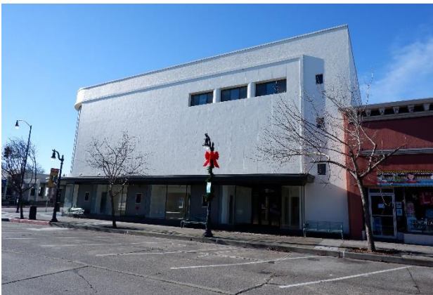
Figure 5. East façade, looking west, showing largely unfenestrated upper two stories framed by a narrow, projecting band.
