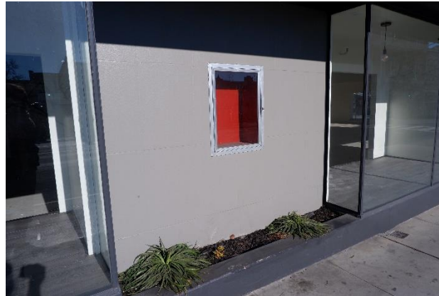
Figure 4. Typical inset display case in the stucco wall between storefront windows.
