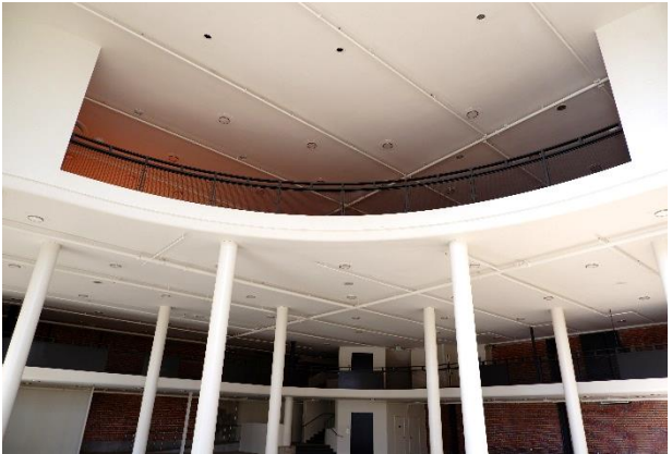
Figure 9. Mezzanine and second story, looking northwest.
