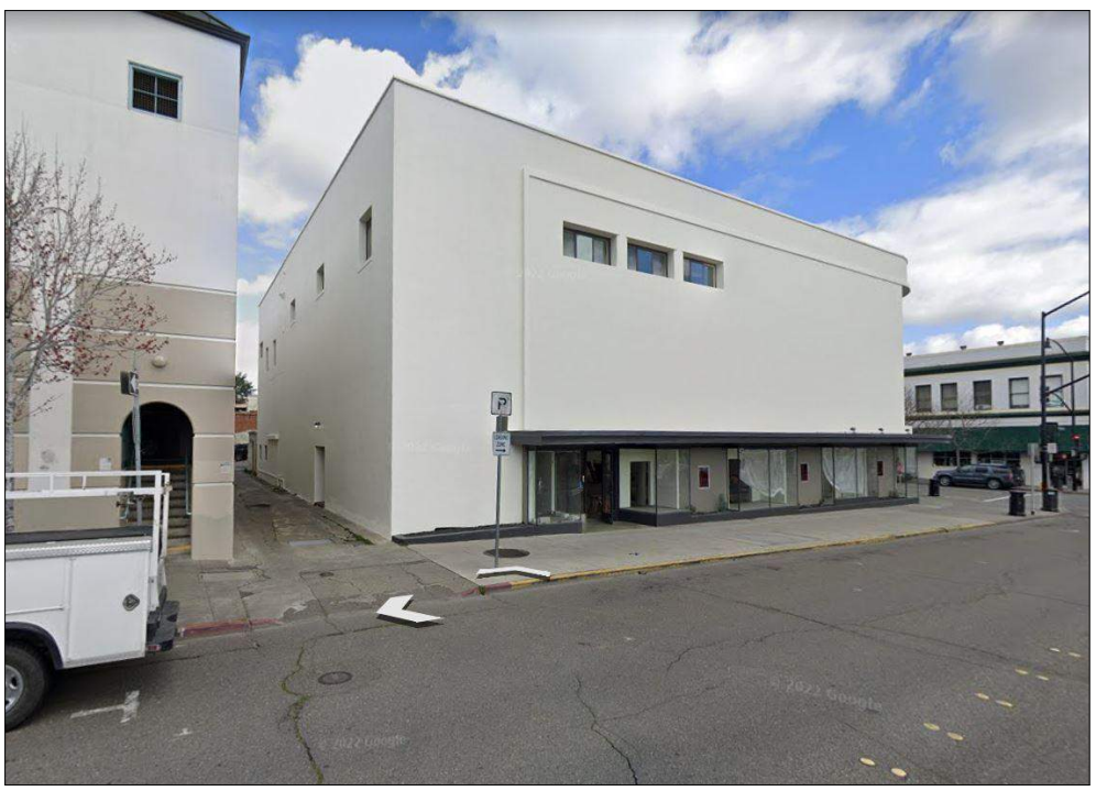
WESTERN AVE & TELEPHONE ALLEY 4
