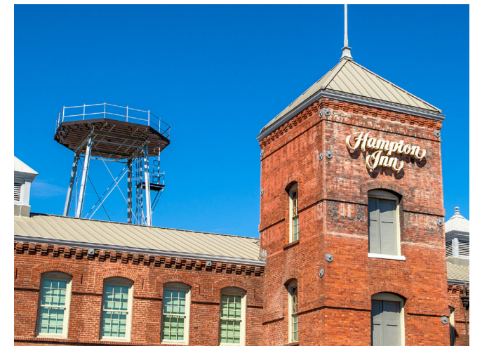
EXISTING METAL ROOF NEW ROOF TO MATCH COLOR & SPACING OF RIBS - VERIFY SAMPLE PRIOR TO INSTALL
