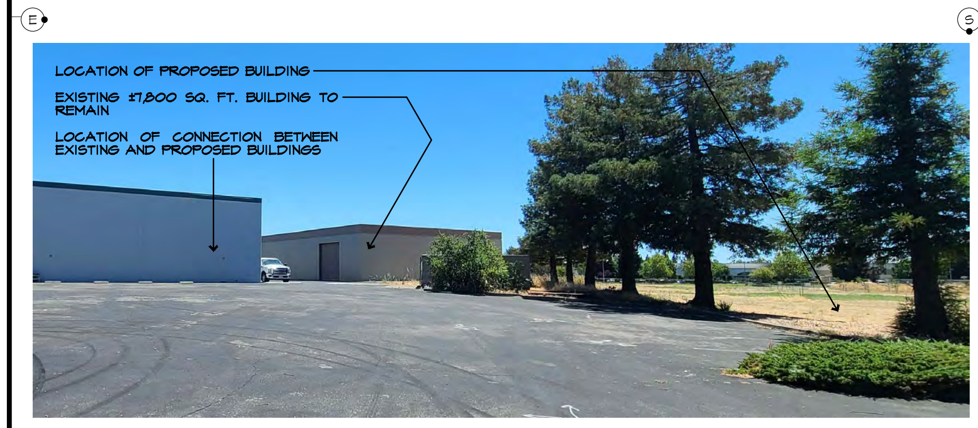
2 SITE PHOTO TAKEN @ (E) WESTERN PARKING AREA FACING SOUTHEAST TOWARDS PROPOSED CONNECTION TO (E) BUILDING
