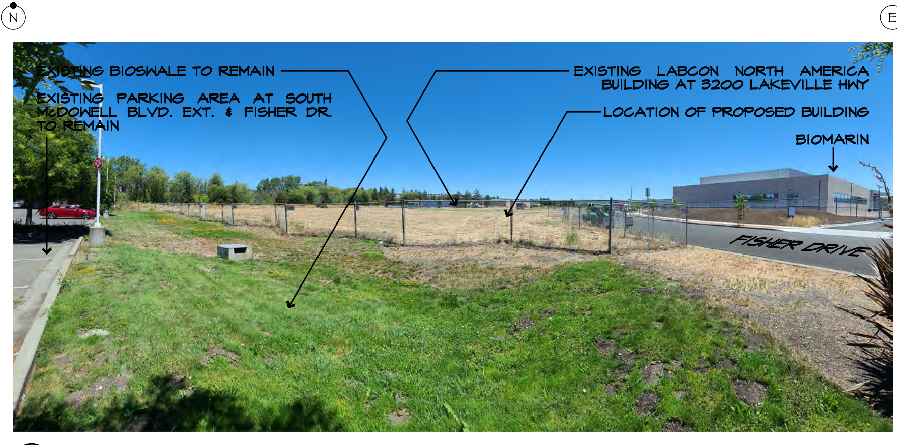
5 PANORAMIC SITE PHOTO TAKEN @ (E) SOUTHWESTERN PARKING AREA FACING NORTHEAST
