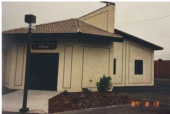
Immediately after 1987 remodel and expansion. Source: Sonoma-Marín Fair Archives.
