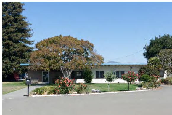
Administration Building in 2021.
