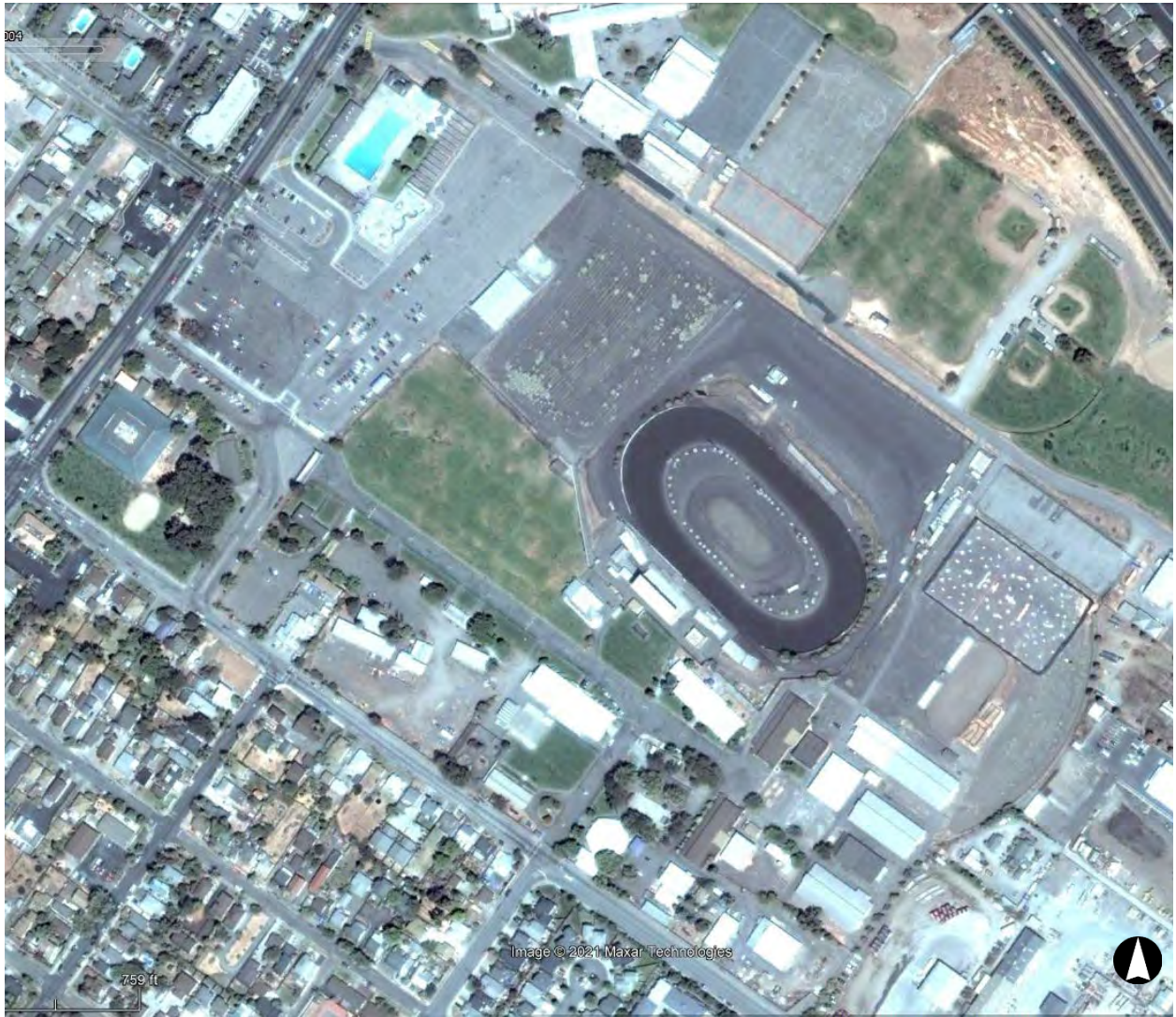
Figure 59. Aerial photograph of the Sonoma-Marin Fairgrounds, August 11, 2004. Source: Maxar Technologies via Google Earth.
