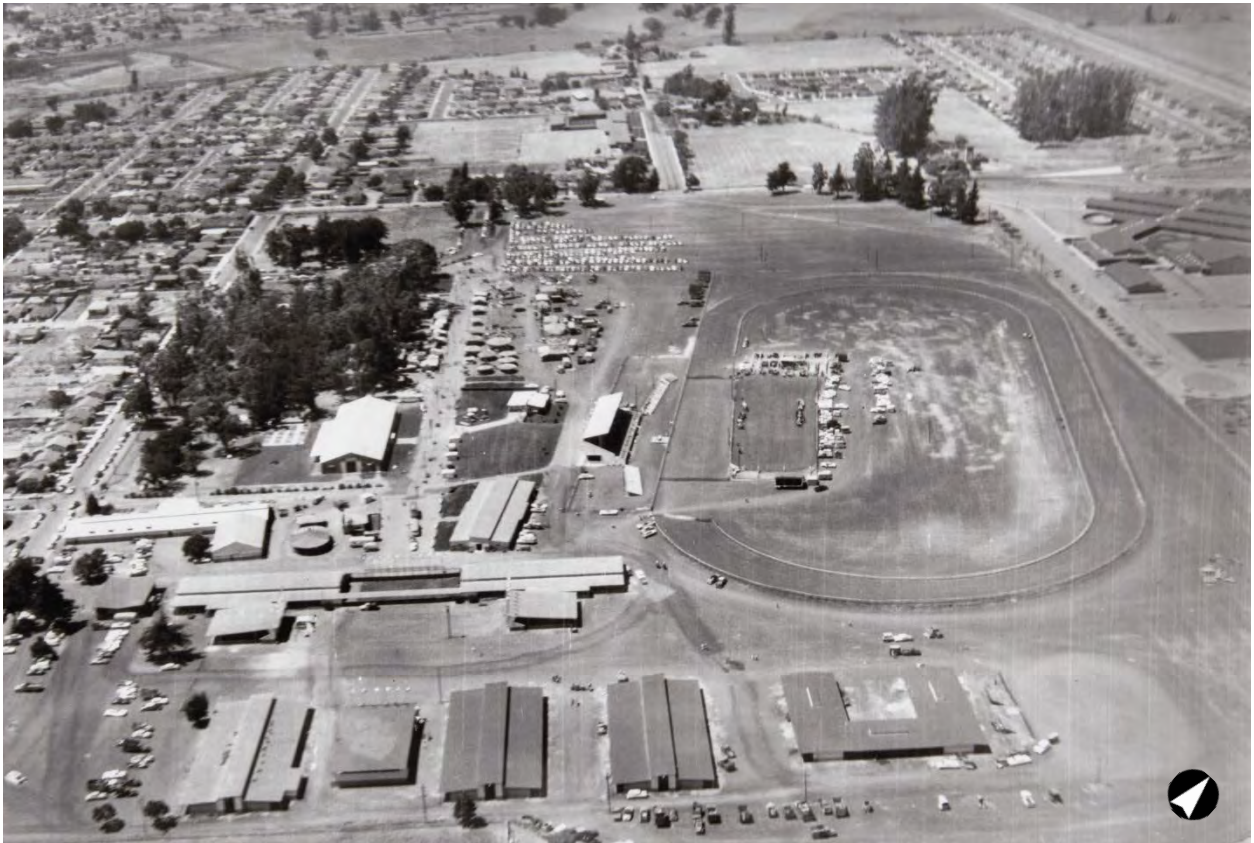
Figure 49. Bird's-eye aerial photograph of the Sonoma-Marín Fairgrounds, circa 1956-58, looking toward E. Washington Street. Note that the Main Exhibit Hall and Gardenway Stage have been constructed and that the Arts & Crafts Building has yet to be erected. Source: Sonoma County Library Digital Collections.
