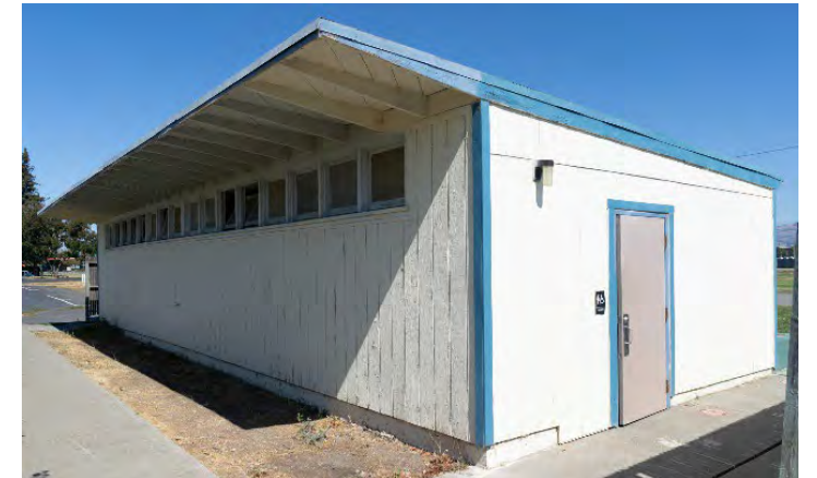
Restroom (Restroom 1), built c. 1953.
