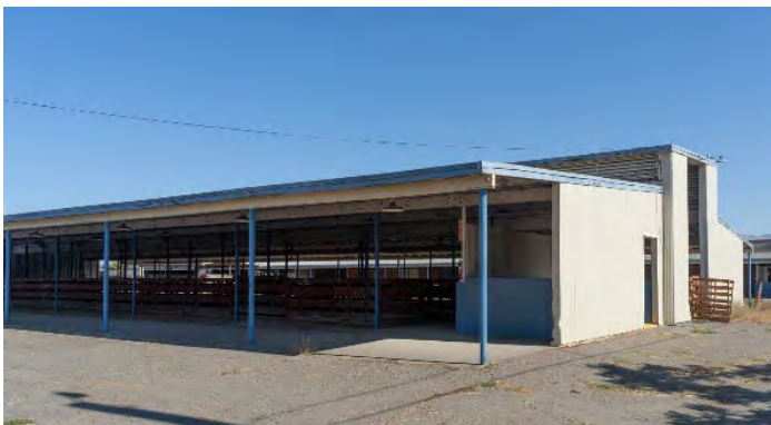
Cattle Barn 2 (Barn 2), built 1948-49.
