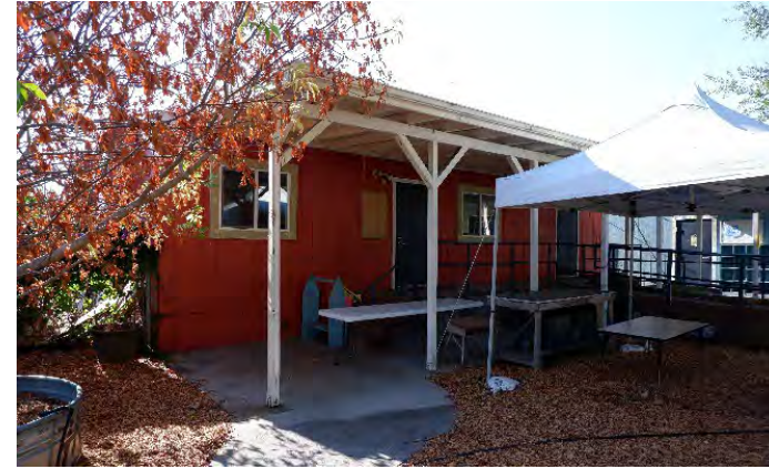
Classroom Modular Building (Live Oak – Classroom 5), built 2004.
