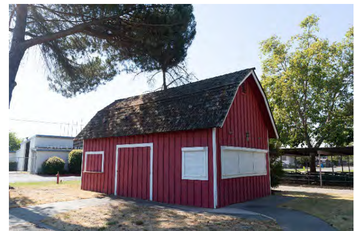
Red Barn, built c. 1965-68.
