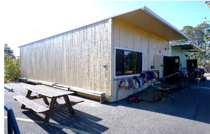
Classroom Modular Building (Live Oak – Classroom 7), built 2013.
