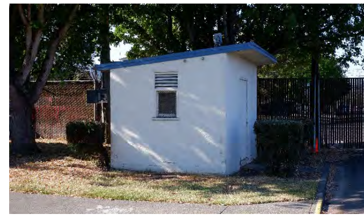
Pumphouse, built c. 1963-65.
