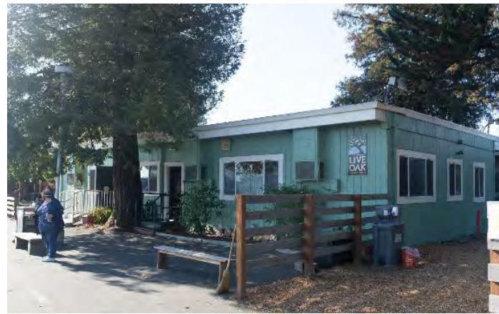
Classroom/Admin Building (Live Oak – Classroom 1), built 1979.
