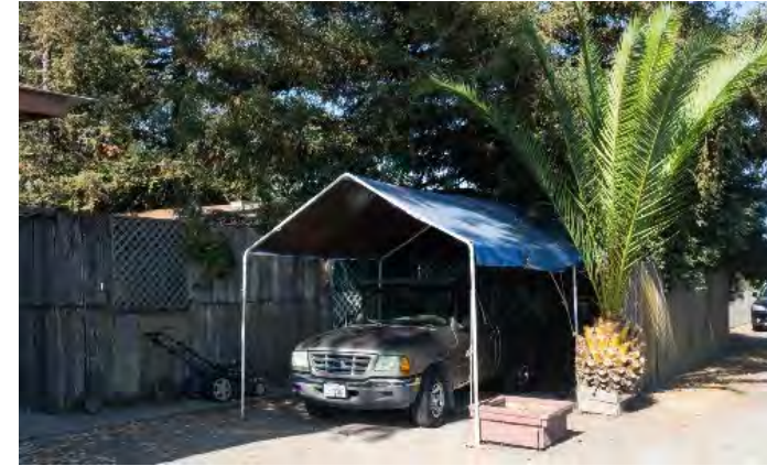
Maintenance Mobile Home, built 2004.
