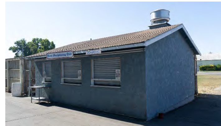
Grandstand Concession (Concession 2), built 1988.
