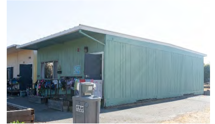
Classroom Modular Building (Live Oak – Classroom 6), built 2008.
