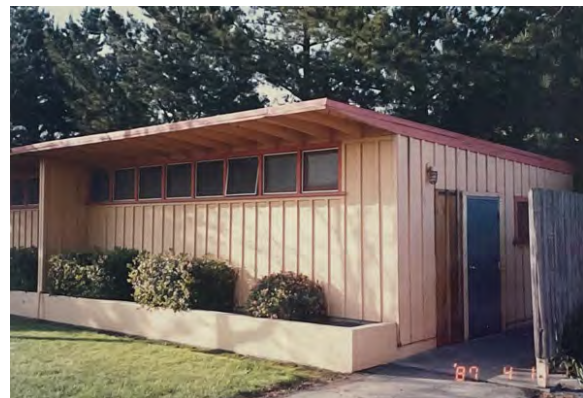
Restroom 2 in 1987. Source: Sonoma-Marín Fair Archives.
