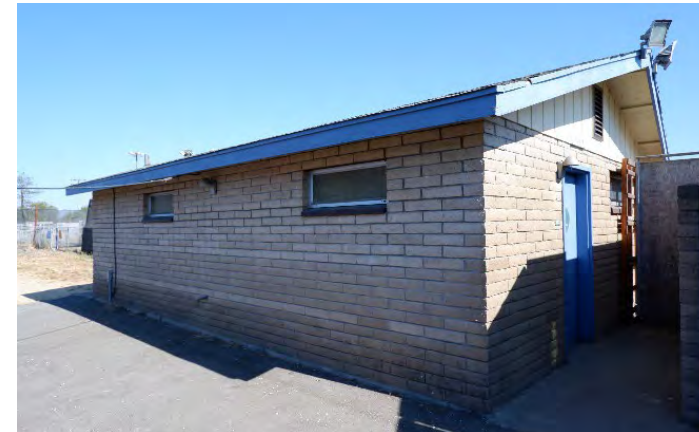
Barn Area Restroom (Restroom 5), built 1974.
