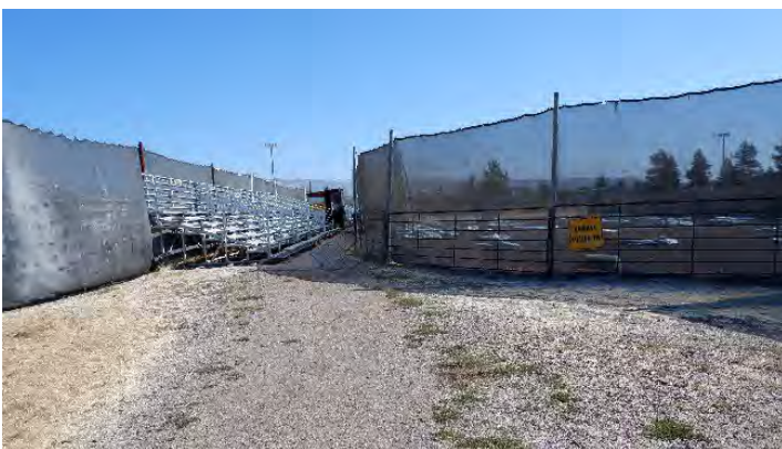
Horse Arena, built c. 1993-2004.
