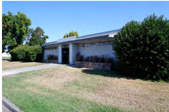
Poultry Building in 2021.
