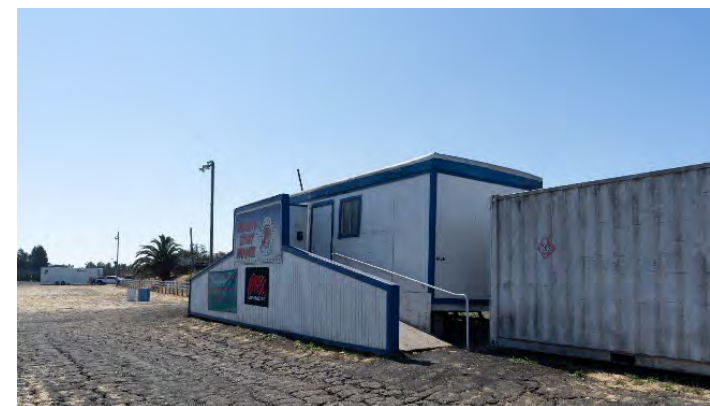
Restroom (Speedway East) (Restroom 6), built c. 1993-2004.
