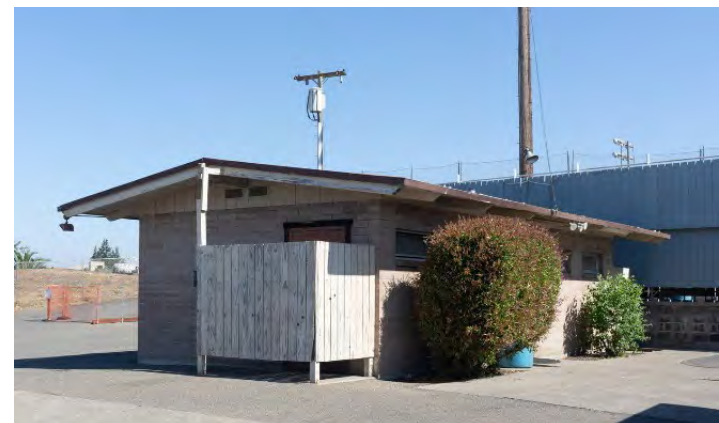
Grandstand Restroom (Restroom 3), built 1962.
