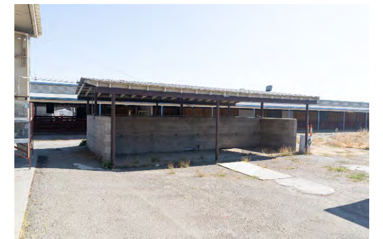
Wash Rack, built c. 1968-73.
