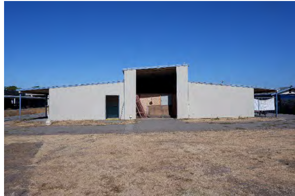
East façade of Cattle Barn 1 in 2021.
