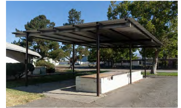
BBQ Pit, built c. 1974.
