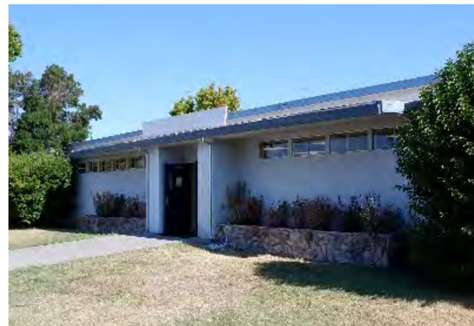
Poultry Building – Community Building, built 1951.
