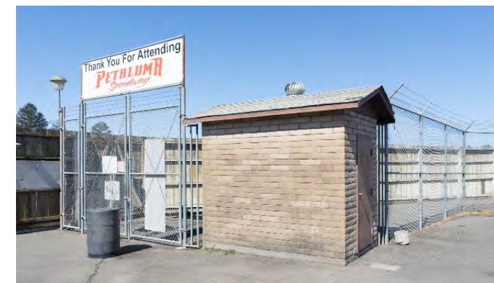
Ticket Booth (Grandstand) (Ticket Booth 2), built c. 1993-2004.
