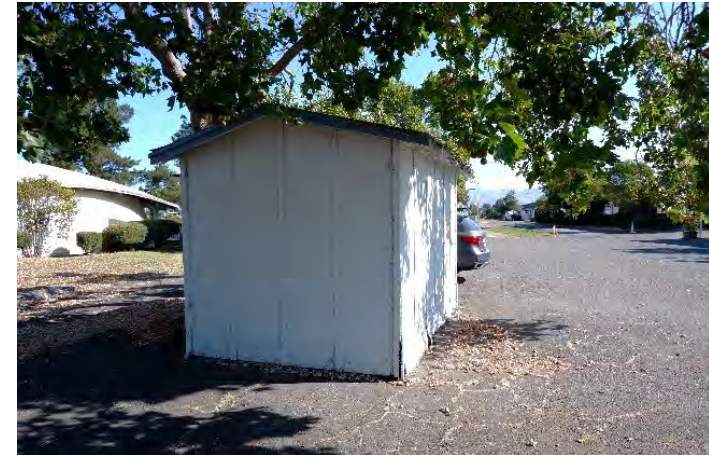
BBQ Pit Storage, built at an unknown date (c. 2010s).
