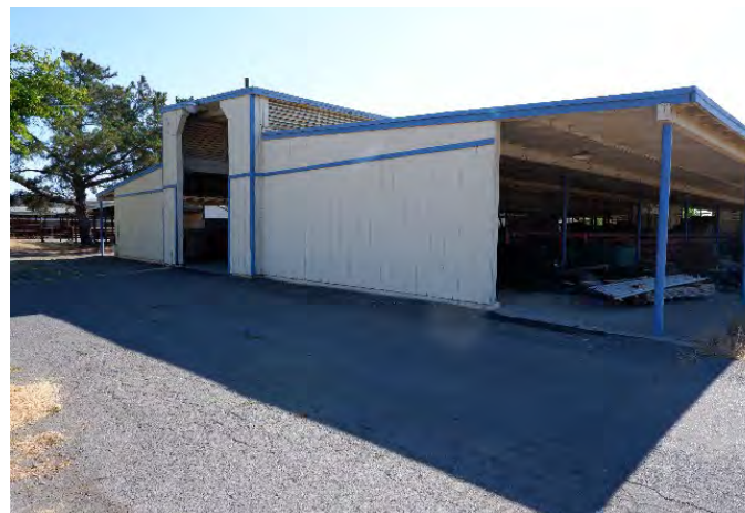
Cattle Barn 3 (Barn 3), built 1950.
