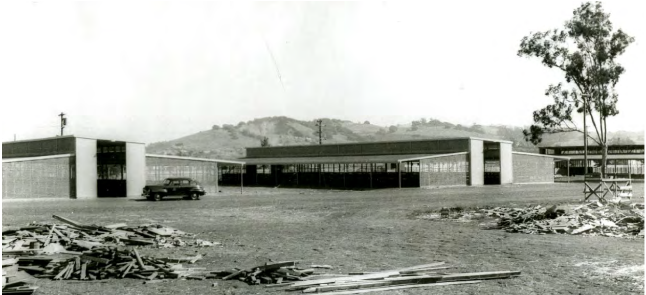
Figure 26. View of all three Cattle Barns in late 1949, while Cattle Barn 3 was still under construction. Source: California State Archives. Department of Public Works (Durkee Collection), F3253: 34
