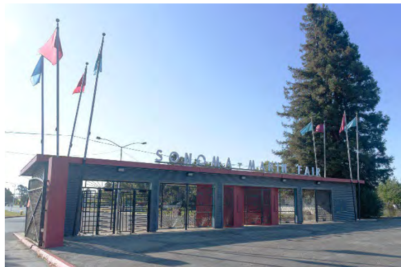
Entrance Gate in 2021.
