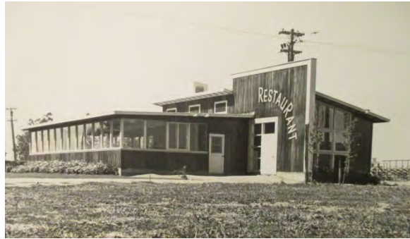
Restaurant soon after 1953 construction. Source: Sonoma-Marín Fair Archives.
