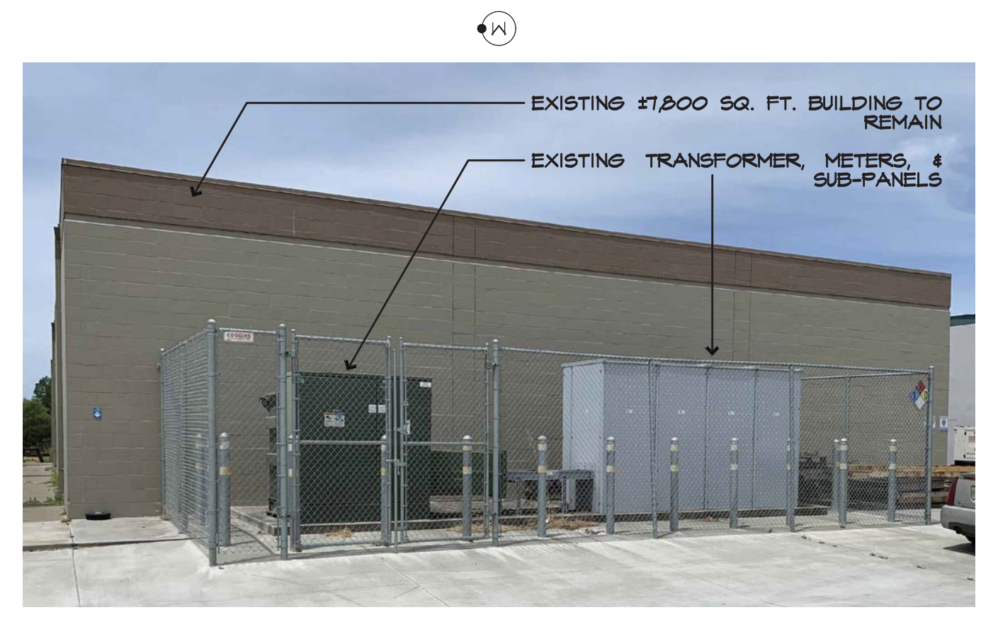
3 SITE PHOTO TAKEN @ (E) SOUTHERN DRIVEWAY AREA FACING WEST
