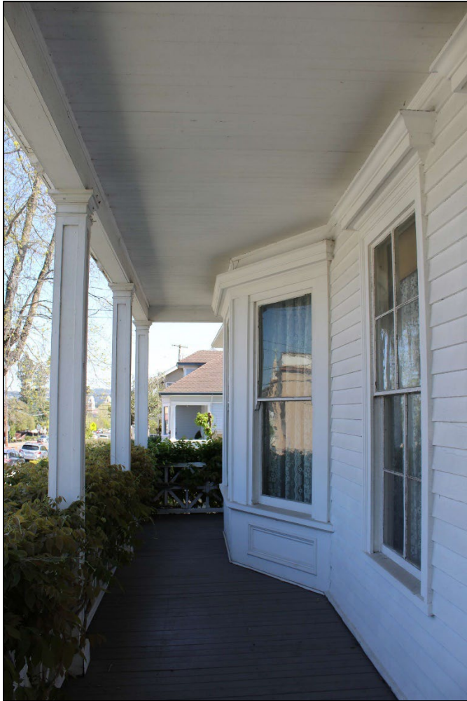
Photo 3 – View of front porch, looking southeast
