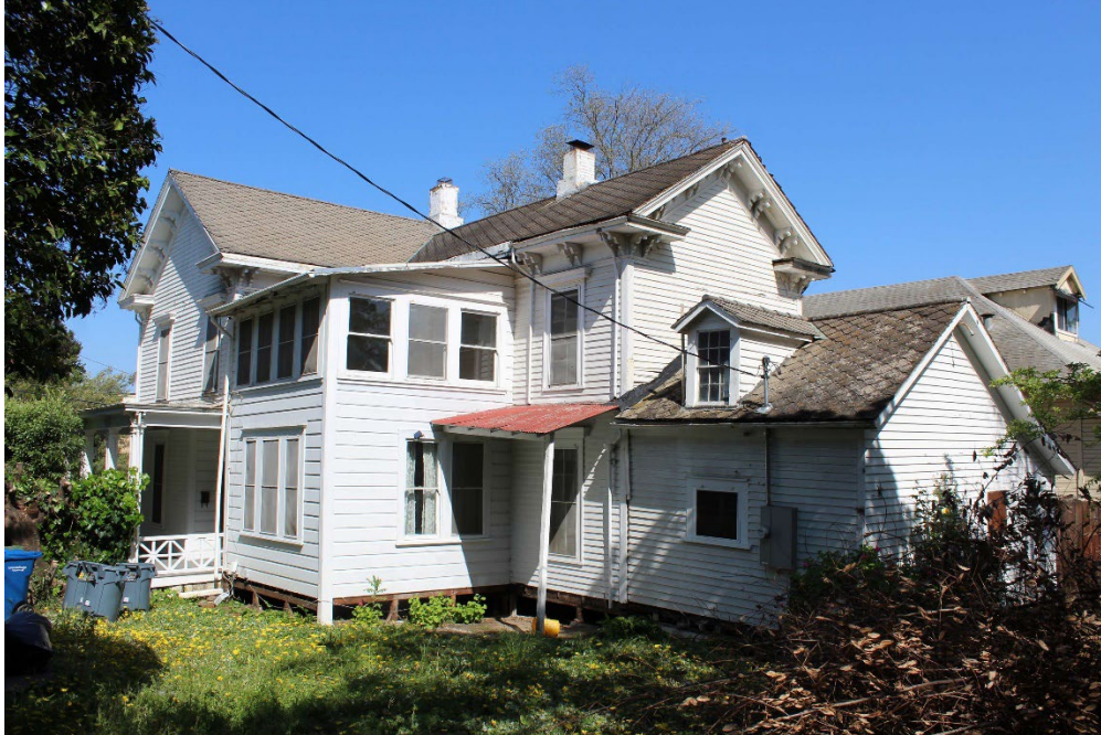
Photo 6 – Northwest side façade, looking northeast
