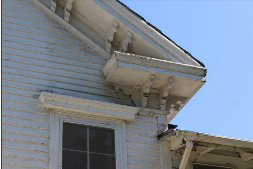
Photo 11 – Eave detail, northwest gable end
