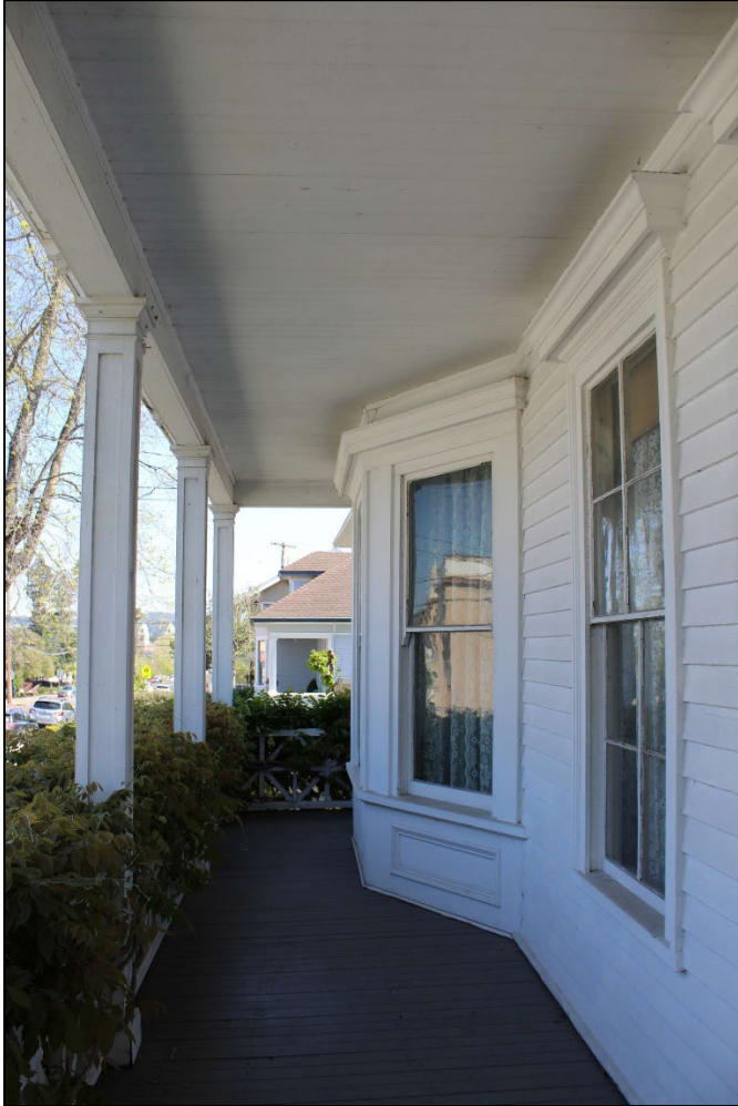
Photo 3 – View of front porch, looking southeast
