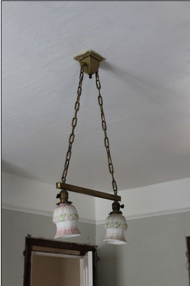
Photo 20 – Interior fixture, typical
