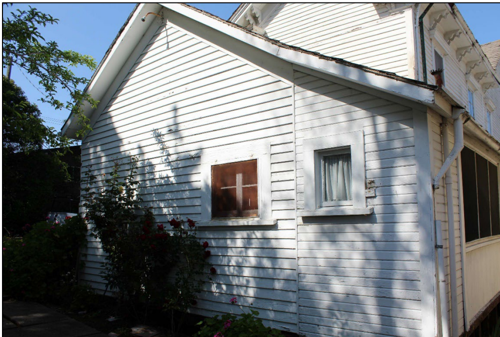
Photo 9 – Rear (southwest) façade, looking northeast
