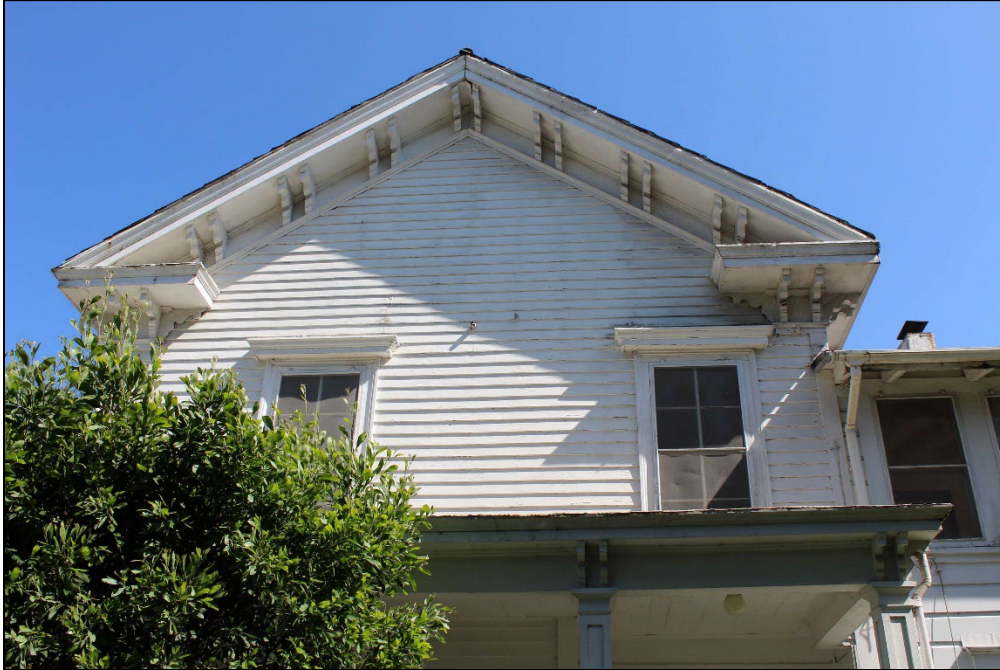
Photo 4 – Northwest gable end
