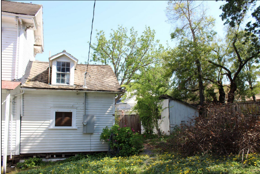
Photo 8 – Rear, one-story addition, looking southeast (shed to right)
