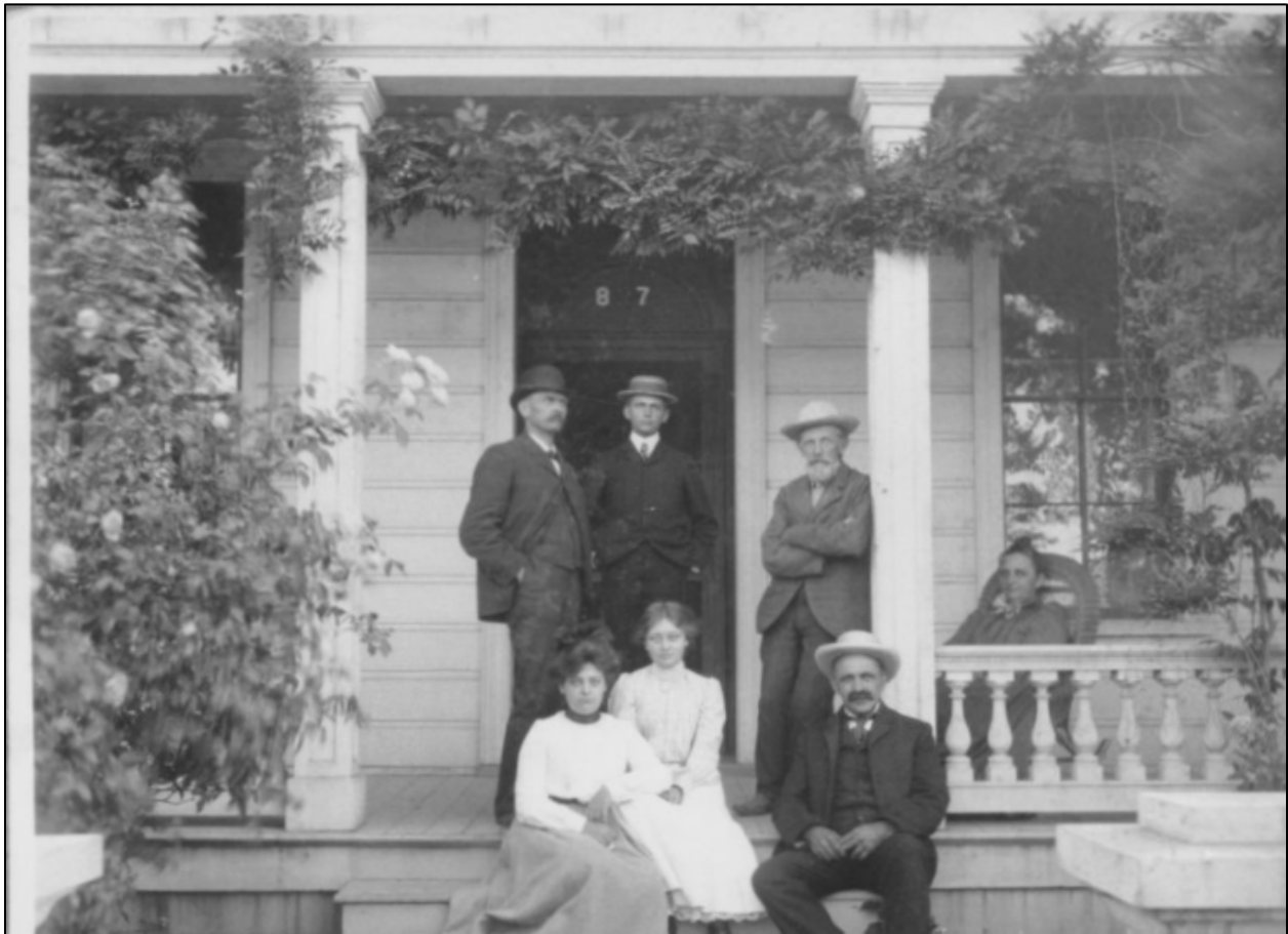
Figure 8 – 245 Howard Street photographed in 1895 with Schluckebier family, when it was on Kentucky Street (note posts on porch, windows, and siding)
