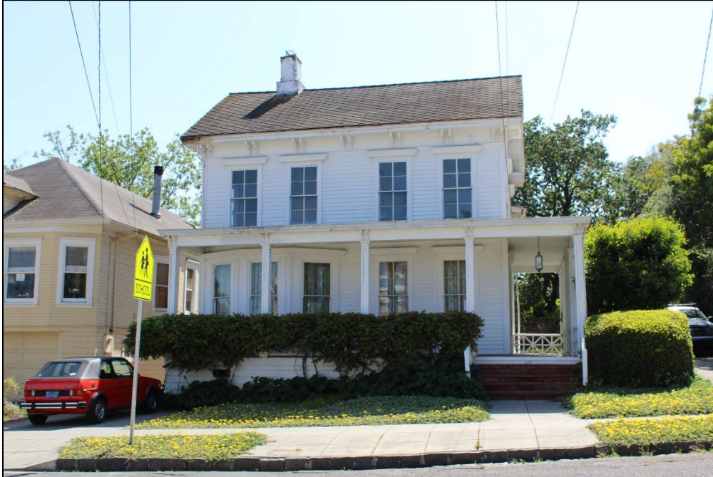
Photo 2 – Front (northeast) façade
