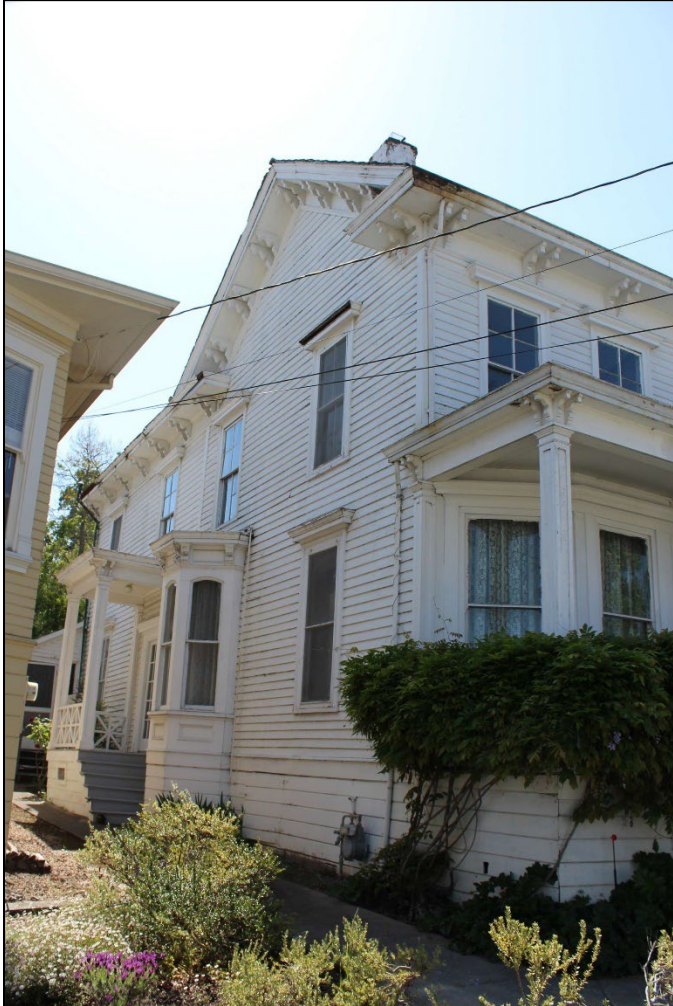
Photo 10 – Southeast side façade, looking southwest
