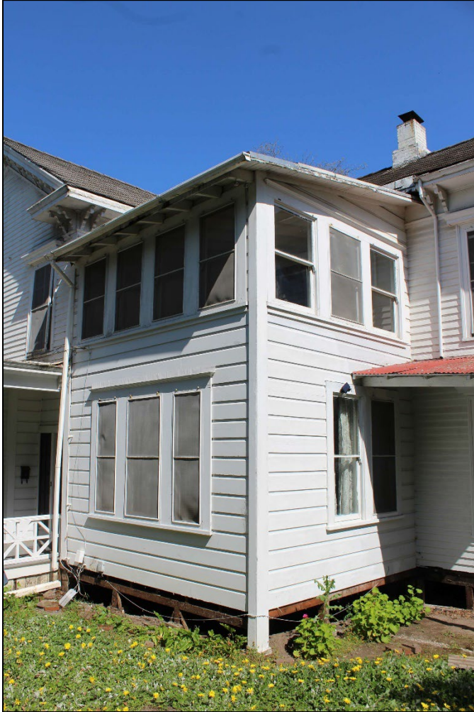
Photo 7 – Sunroom, looking northeast
