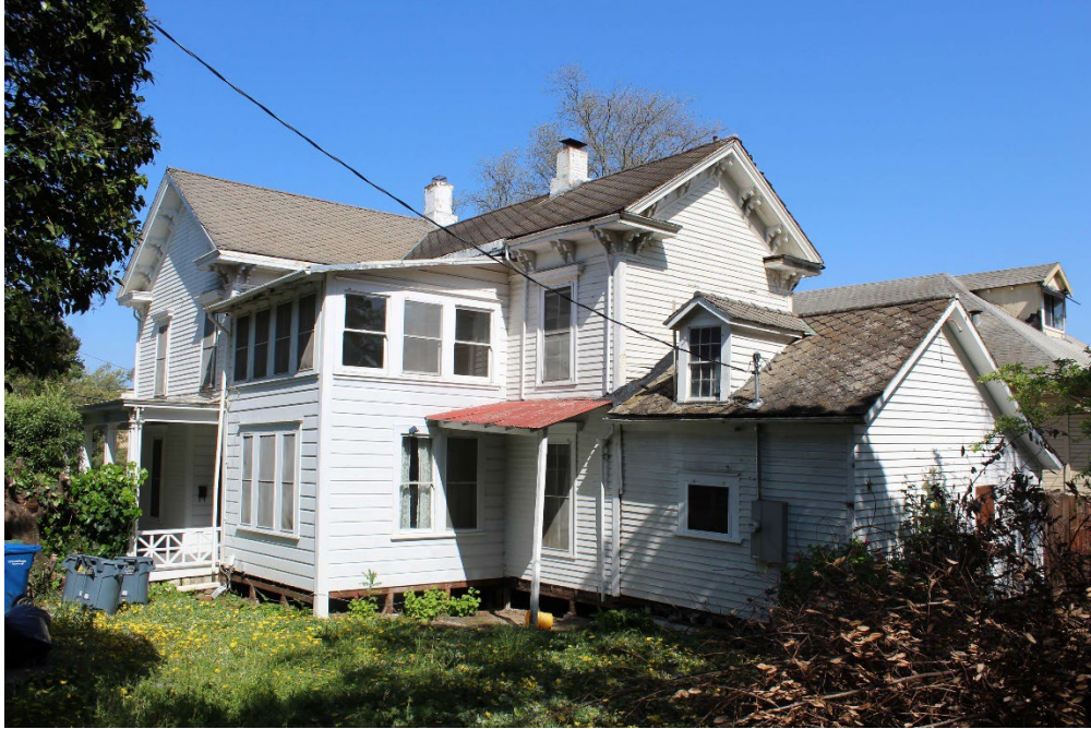
Photo 6 – Northwest side façade, looking northeast
