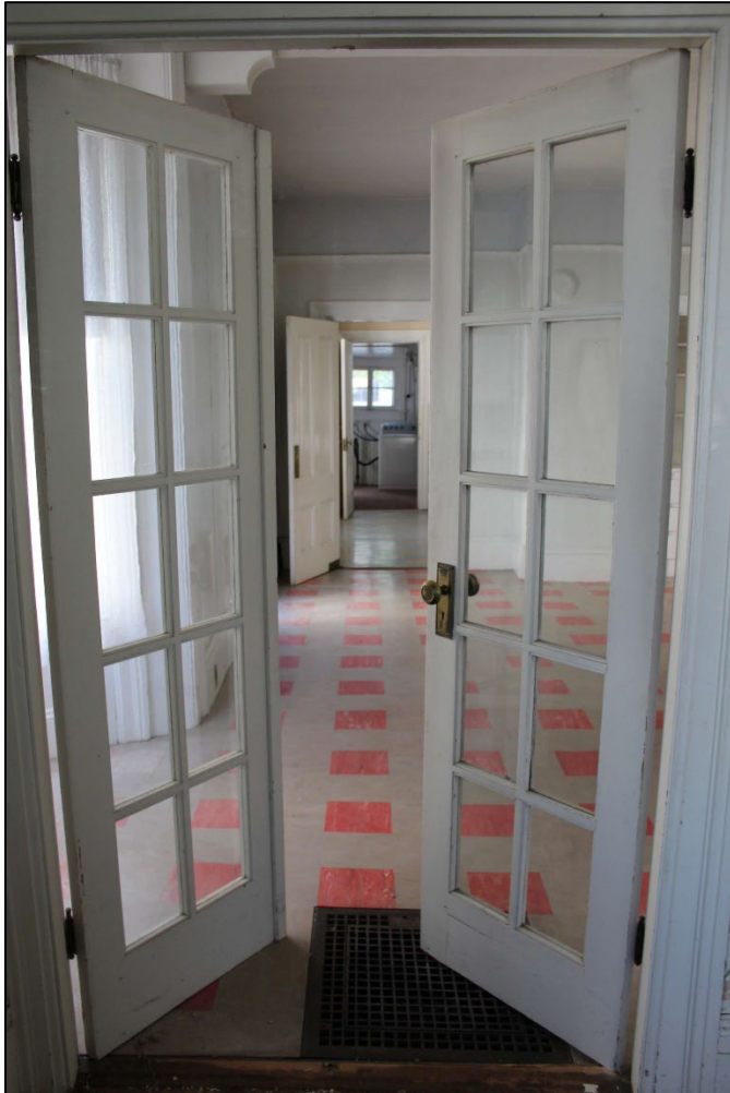
Photo 14 – Looking toward kitchen from living room (looking southwest)
