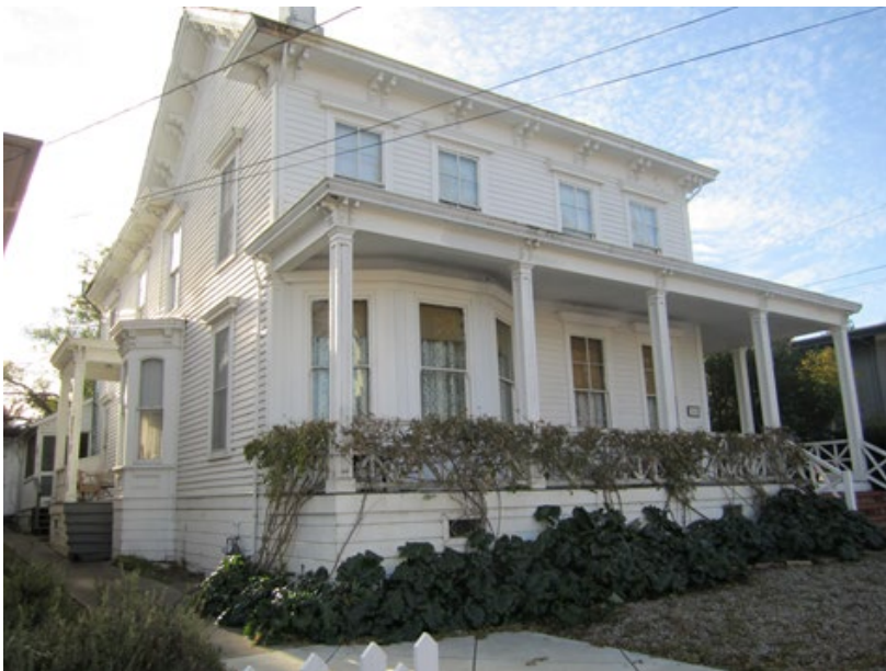
View of SE façade. Photo taken 12.16.13
