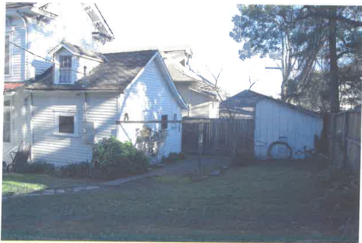
REAR ADDITION TO HOUSE AS SEEN FROM REAR YARD
