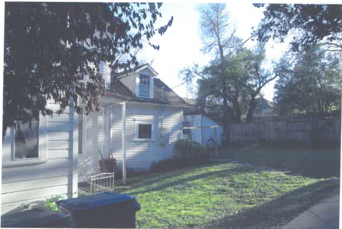
REAR RIGHT SIDE HOUSE
