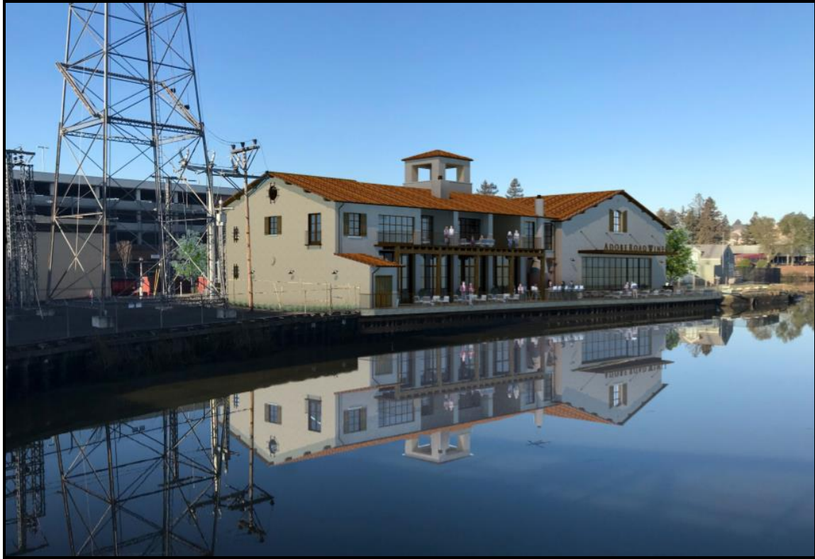
Figure 5: View from the D Street Bridge
