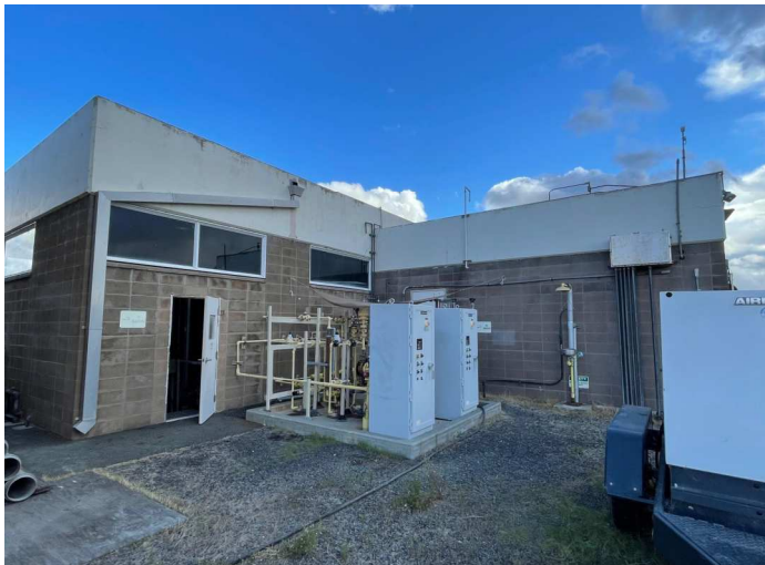
Photo 5: Hypochlorite and Bisulfite pumping area
