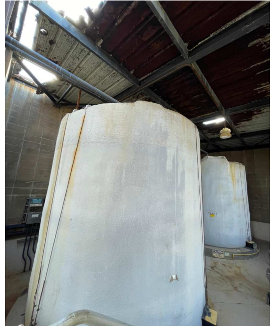
Photo 4: Two Sodium Bisulfite tanks inside existing building
