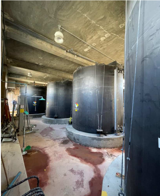
Photo 3: Four Sodium Hypochlorite tanks inside existing building
