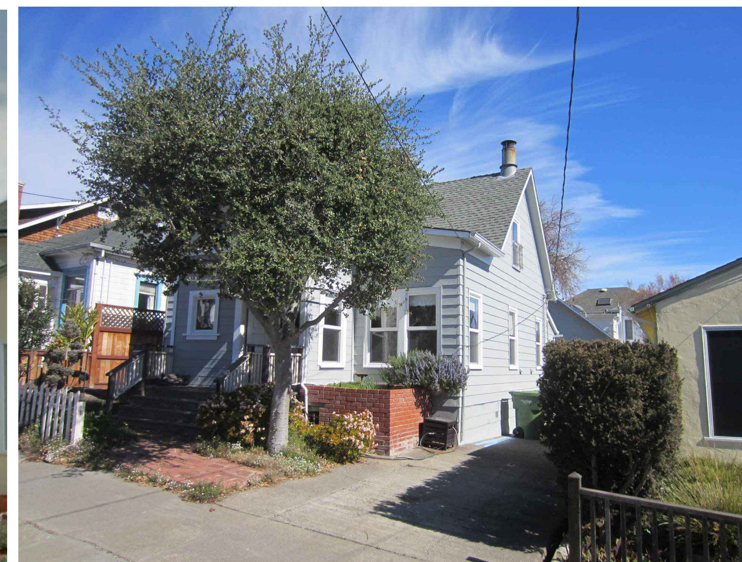
FRONT ELEVATION FROM SOUTHWEST
