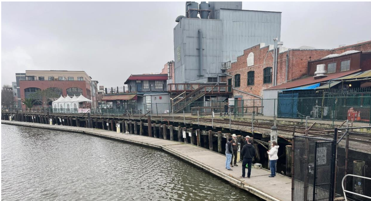
Figure 1. Consulting engineers and timber scientists met on December 22, 2022 to evaluate and plan the logistics for a detailed assessment of every timber member, which will inform decisions about design, costs of construction, ownership, and permits.
