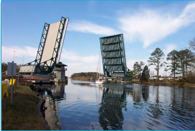
Photo 1 - A dual rolling leaf bascule bridge with overhead counterweight in Chesapeake Virginia of similar span length to that proposed for the Caulfield Lane Bridge over the Petaluma River.
