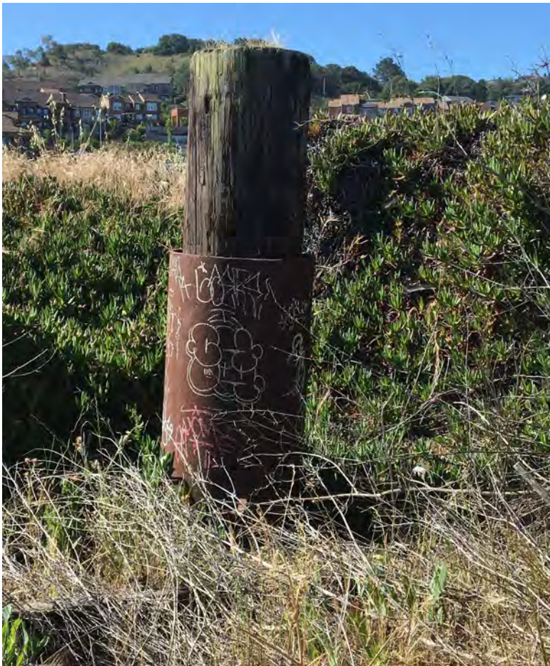
Photograph 1. Iron-encased mooring piling, camera facing south.
