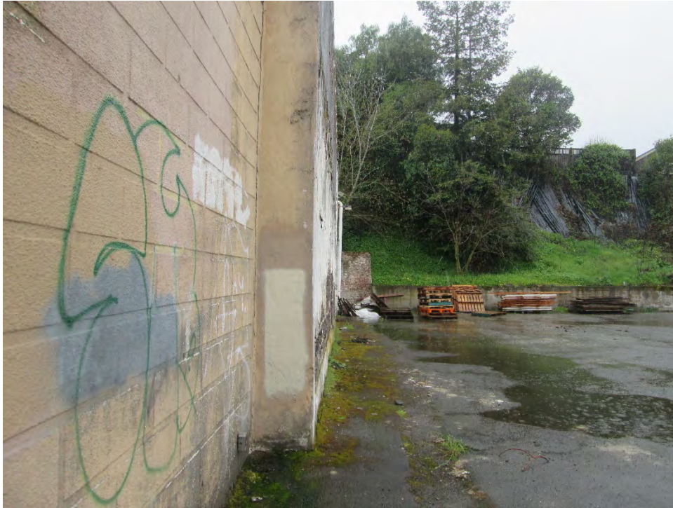
Photo 5: Looking west at the side of the concrete block building
