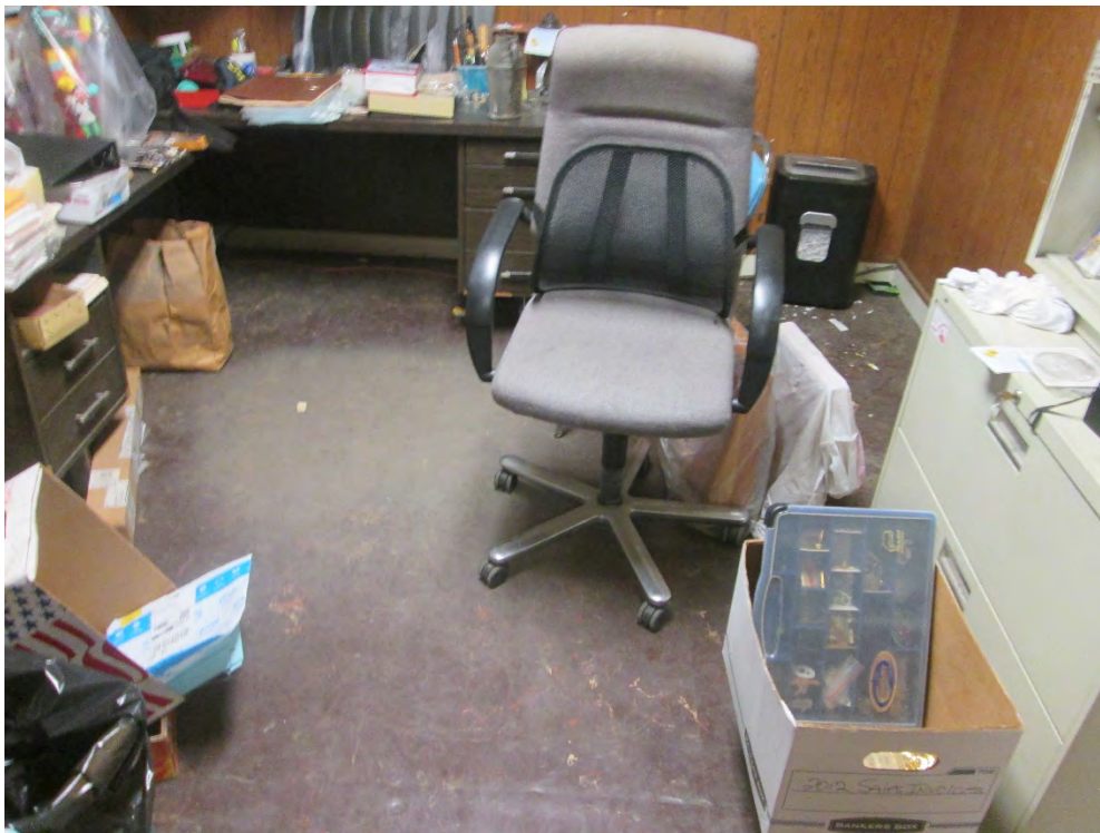
Photo 14: Looking inside the office area within the existing structure
