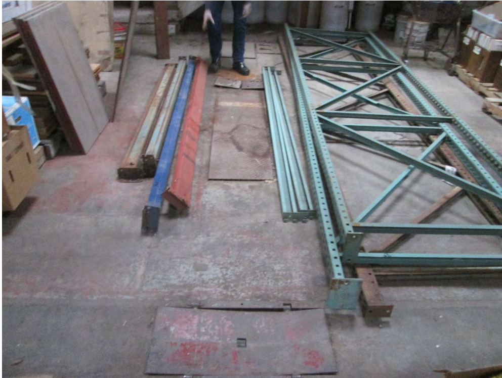
Photo 25: Looking at one of the inground lifts inside the garage structure
