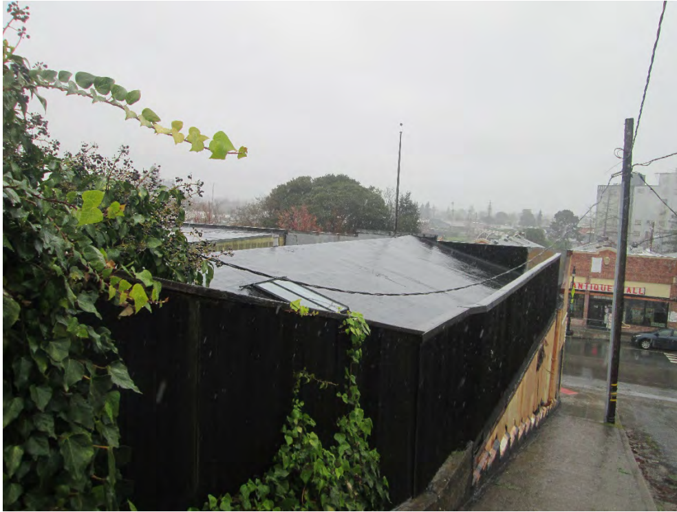
Photo 3: Looking east at the side of the structure from Prospect Street
