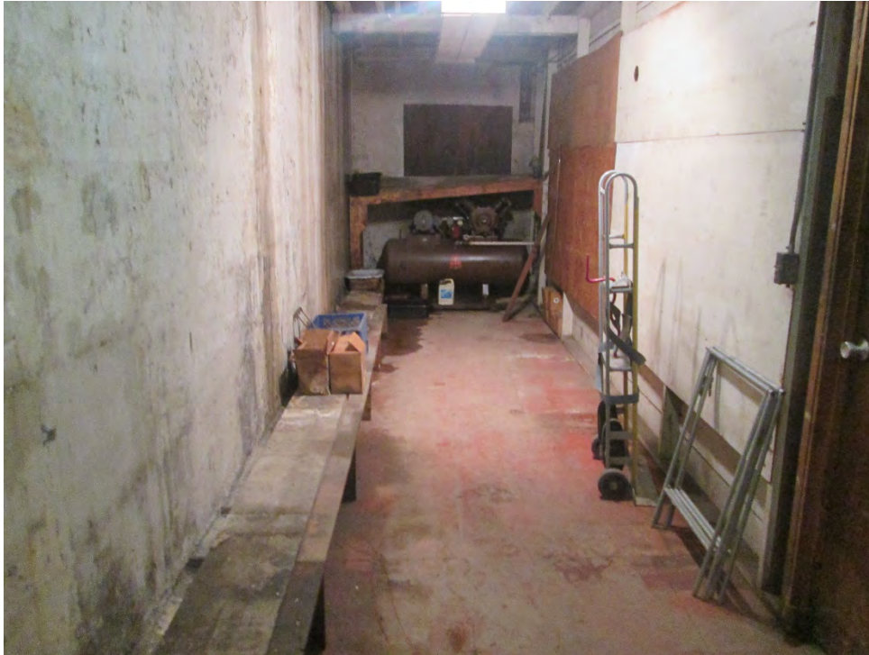
Photo 19: Looking at one of the storage areas inside the garage structure
