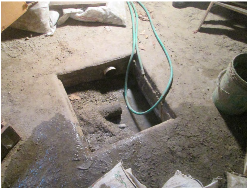
Photo 24: Looking at one of the sumps inside the garage building
