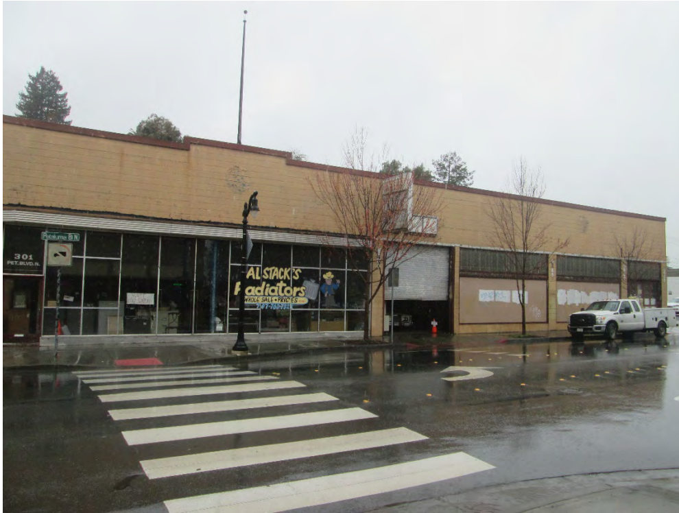
Photo 1: Looking west at the Subject Property
