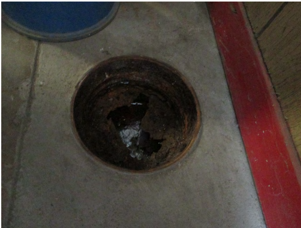
Photo 16: Looking at one of the existing sumps inside the garage structure
