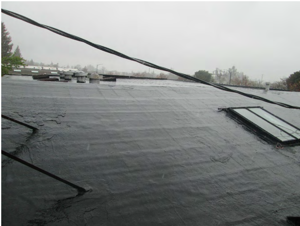
Photo 2: Looking at the ceiling of the existing structure
