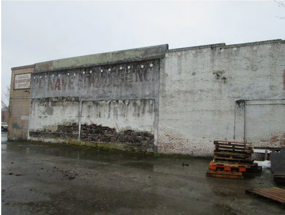
Photo 11: Looking north at side of the existing structure
