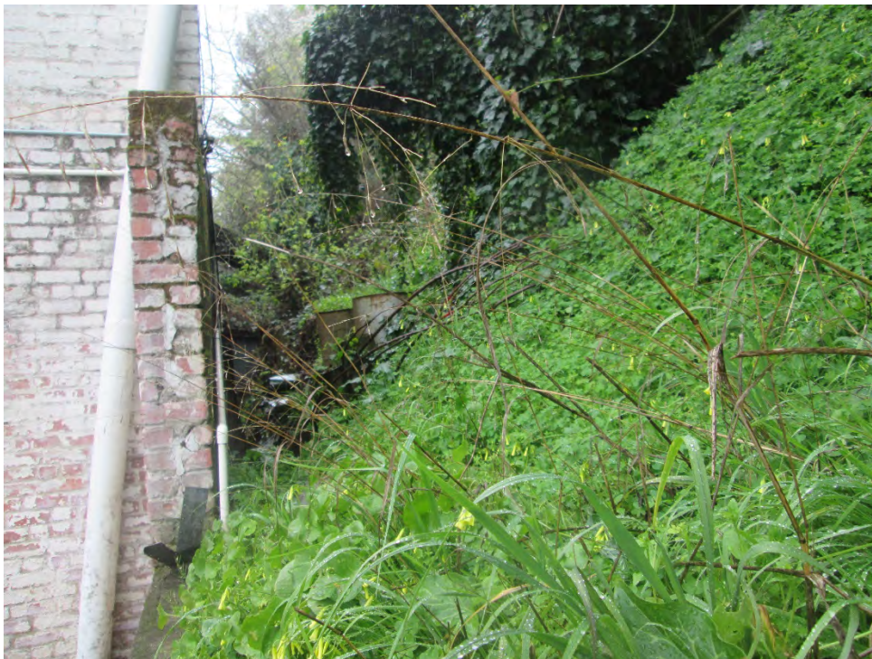
Photo 10: Looking north at the back side of the structure
