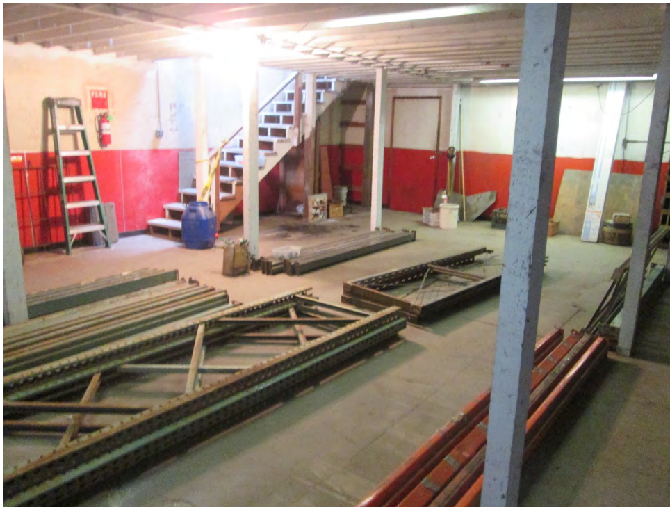
Photo 20: Looking inside the garage structure
