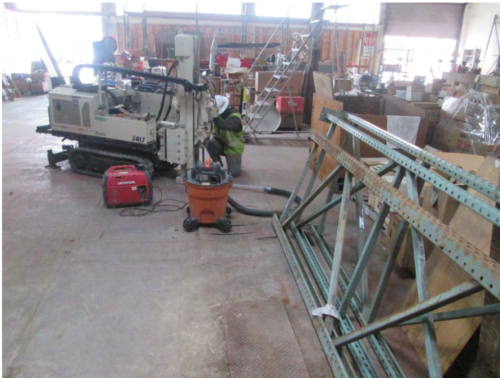
Photo 10: ECA staff drilling at Boring 2 inside the former garage structure
