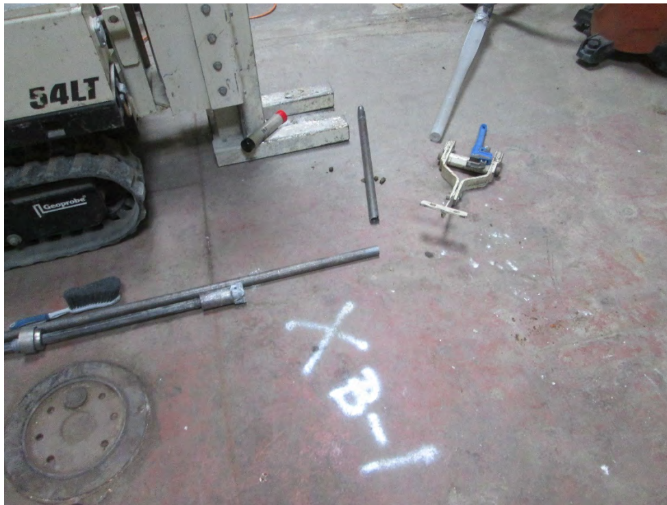
Photo 15: Soil sample at Boring 1 inside the former garage structure
