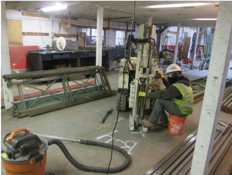
Photo 19: ECA staff drilling at Boring 4 inside the former garage structure
