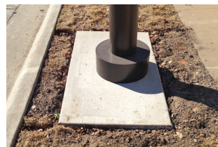
Acceptable Footer Detail
