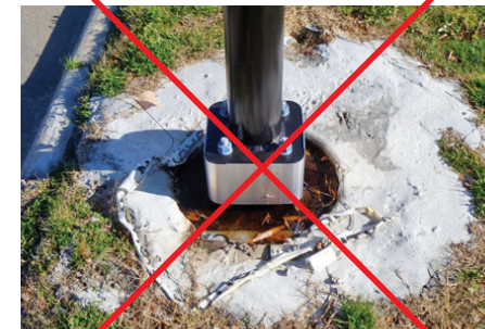
NOT Acceptable Footer Detail
