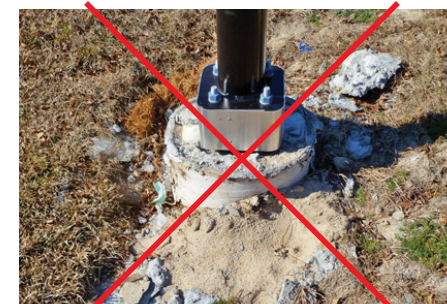
NOT Acceptable Footer Detail
