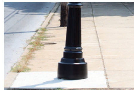
Acceptable Footer Detail
