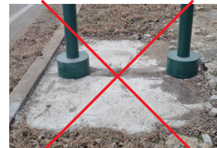
NOT Acceptable Footer Detail
