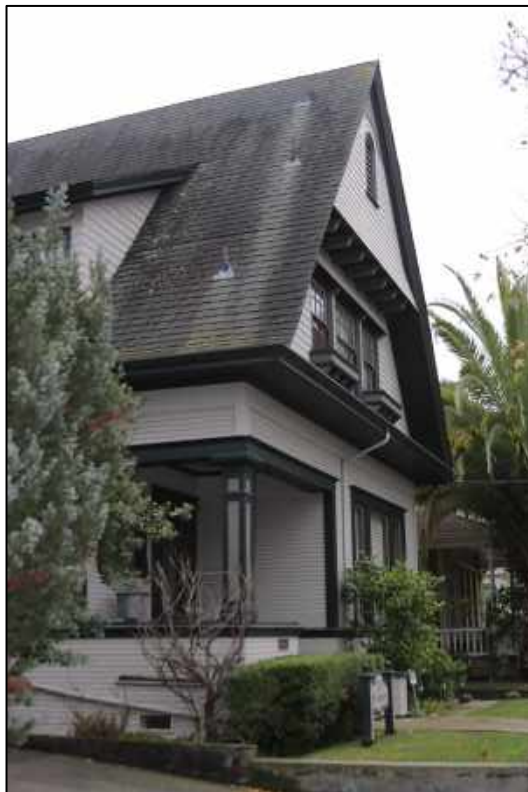
Figure 6: West elevation, porch, northwest corner
