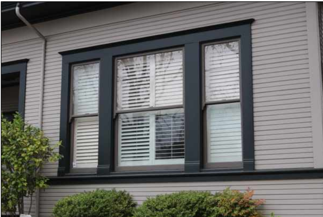
Figure 2: West elevation, tripartite windows
