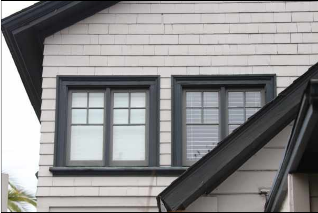
Figure 23: East elevation, upper windows at southeast corner
