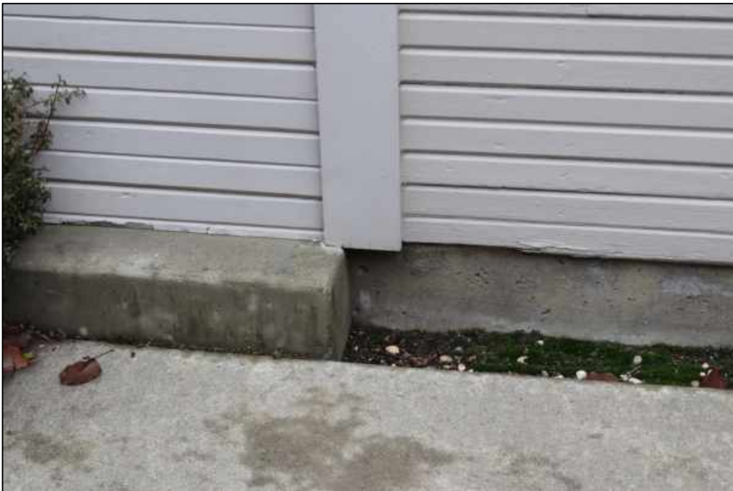
Figure 38: South elevation, foundation
