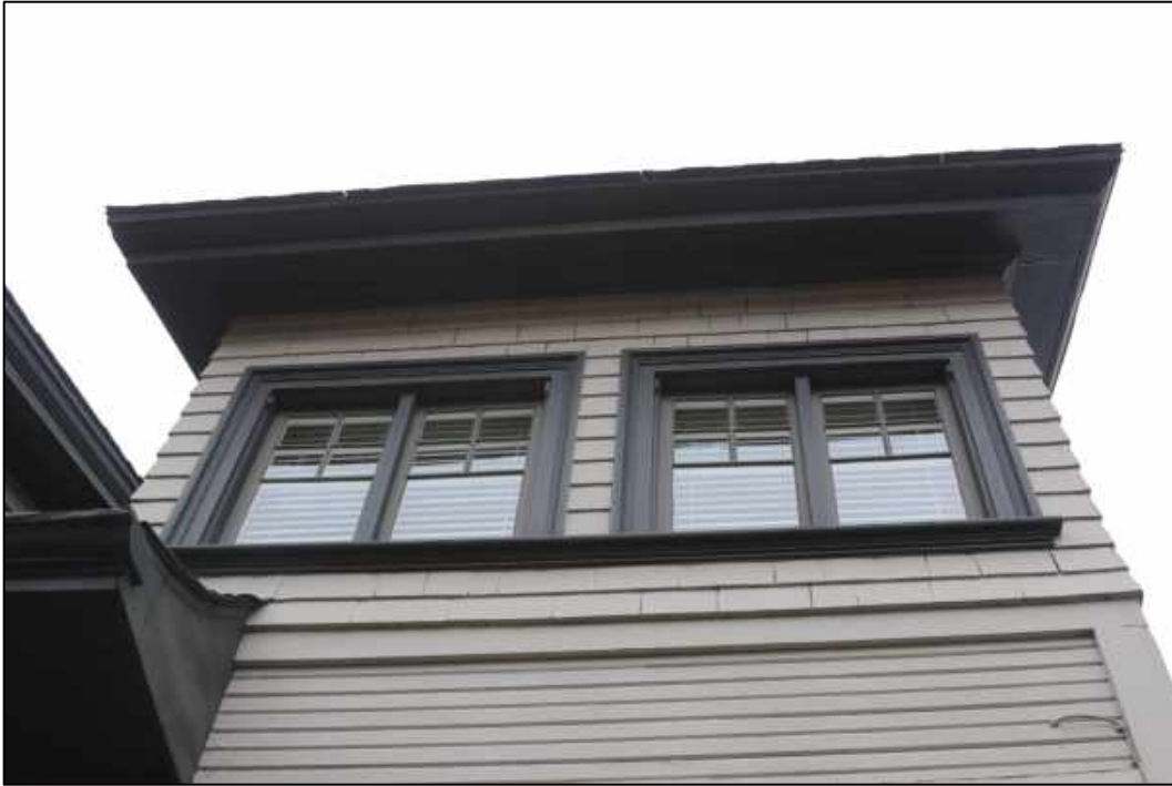
Figure 37: South elevation, upper level windows at southeast corner
