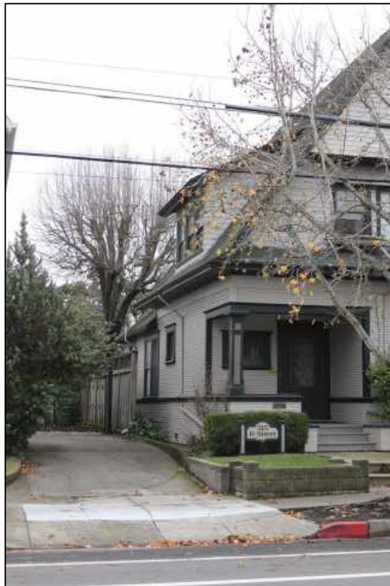
Figure 10: West elevation, northwest corner, neighbor's driveway
