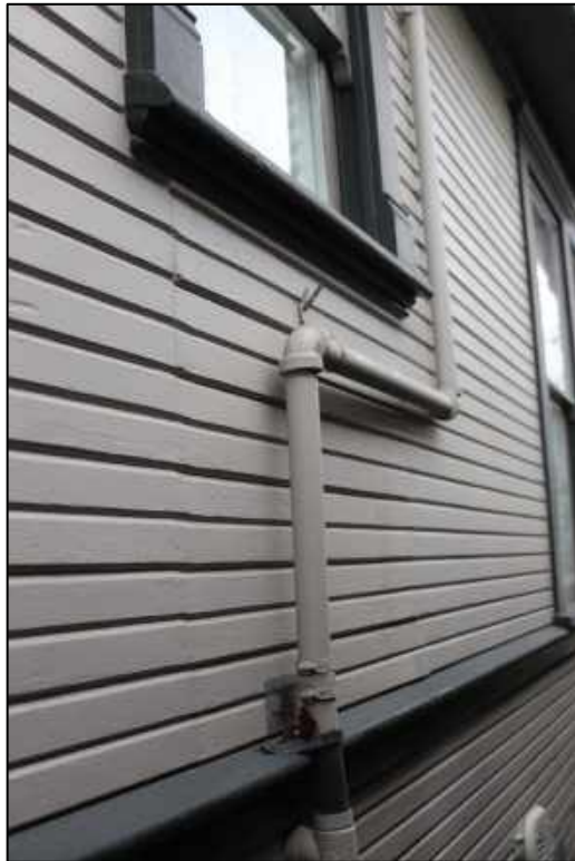
Figure 12: North elevation, patched siding (possible window infill)
