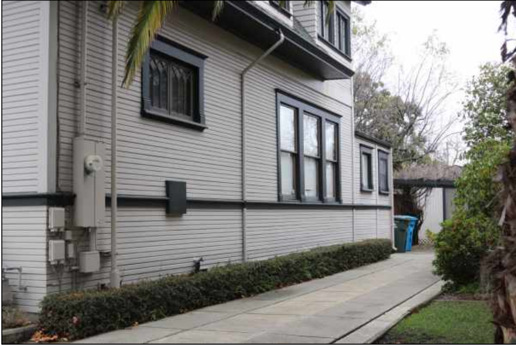
Figure 31: South elevation, lower level, looking east
