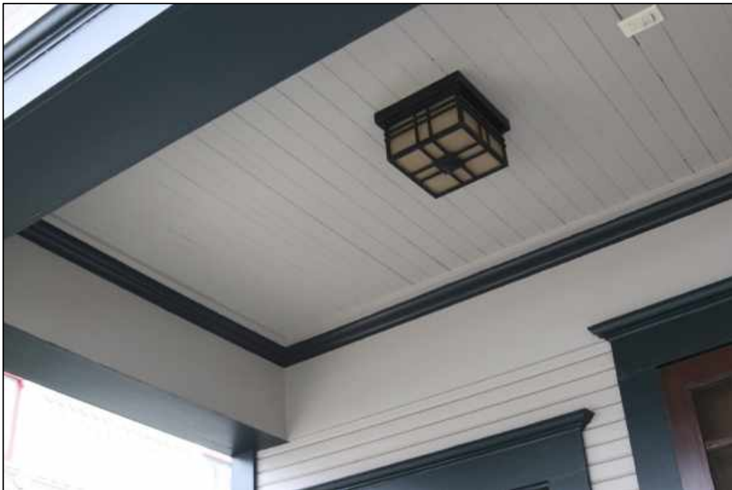
Figure 8: West elevation, porch ceiling
