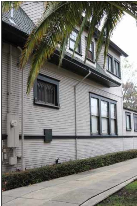
Figure 32: South elevation, looking east
