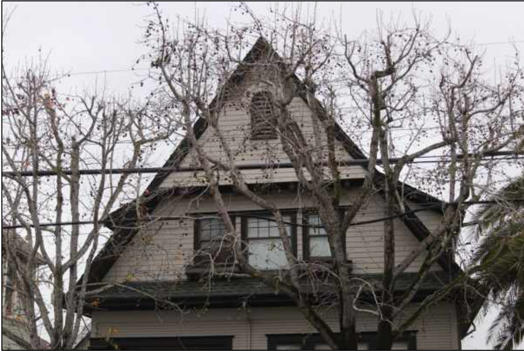
Figure 3: West elevation, upper story
