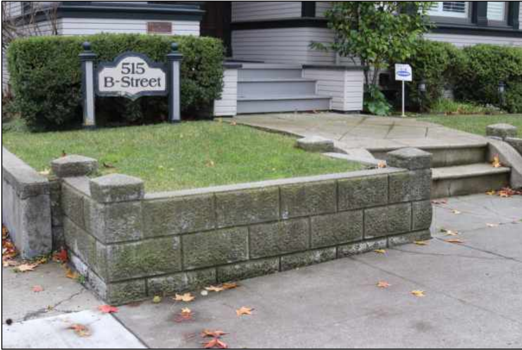
Figure 9: West elevation, retaining wall
