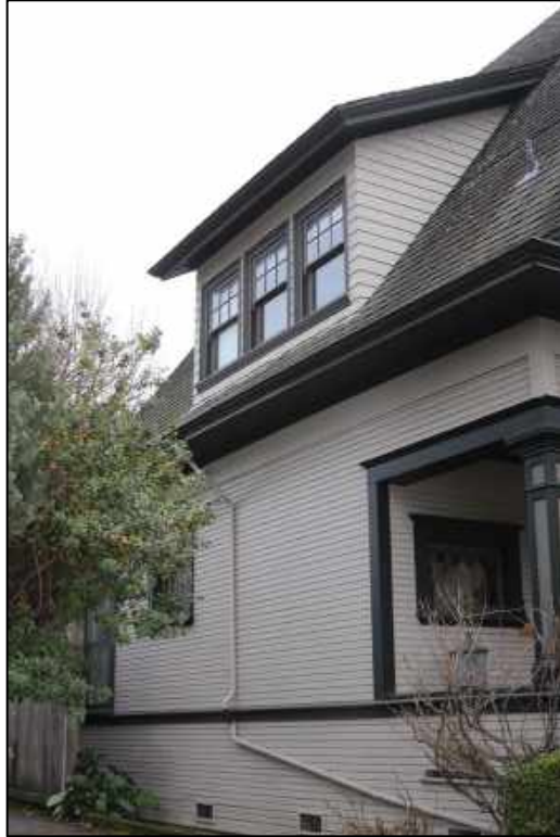
Figure 11: North elevation, shed dormer windows
