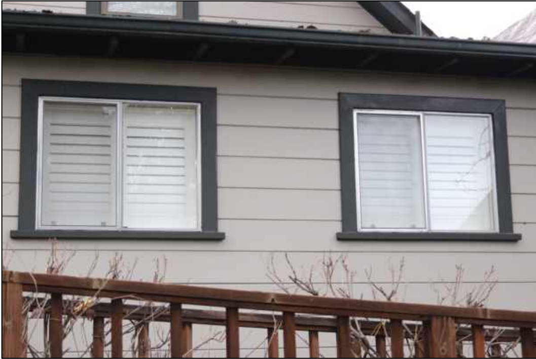
Figure 27: East elevation, modern aluminum sliding windows
