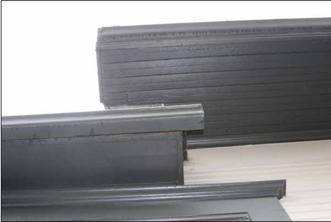
Figure 17: North elevation, eaves
