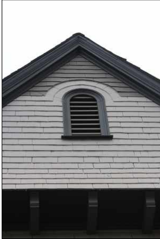
Figure 5: West elevation, vent in gable peak
