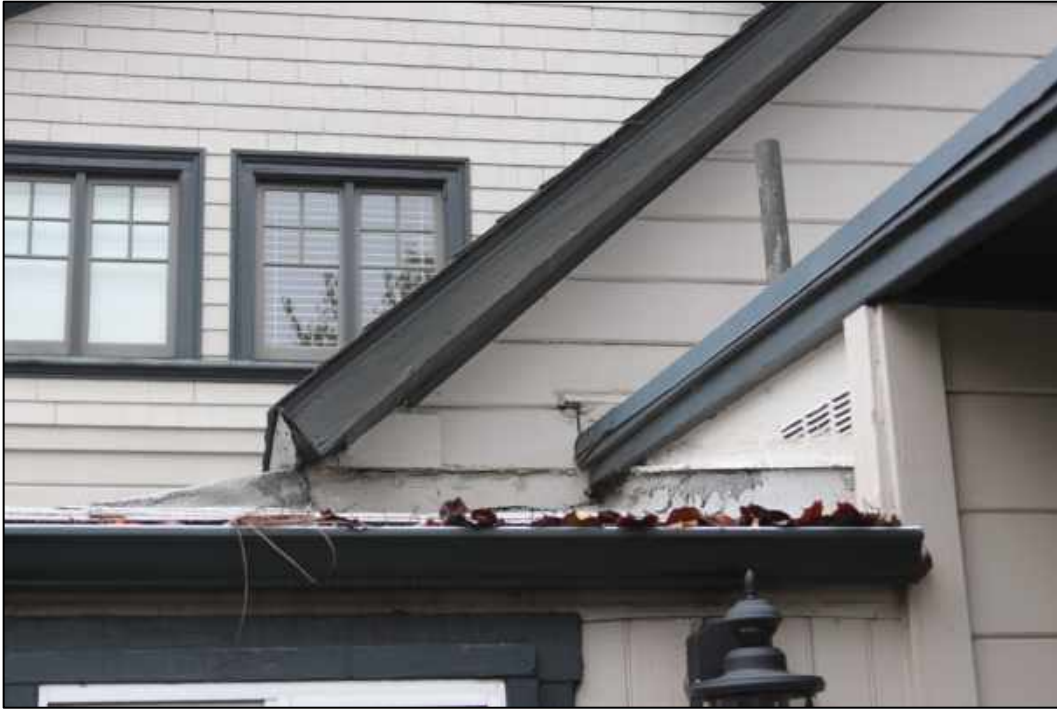
Figure 25: East elevation, fascia boards
