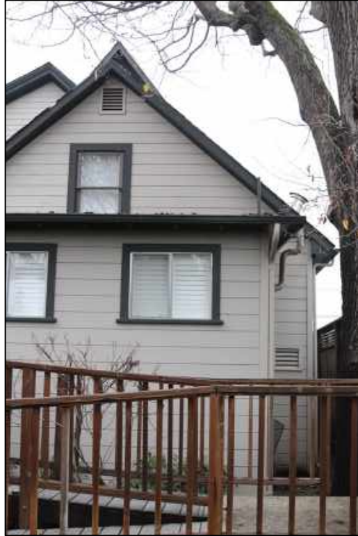
Figure 21: East elevation, shed roof addition and ramp
