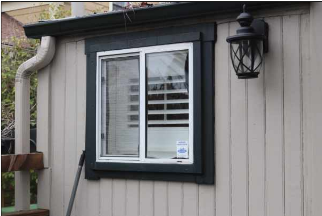
Figure 28: East elevation, modern aluminum sliding window
