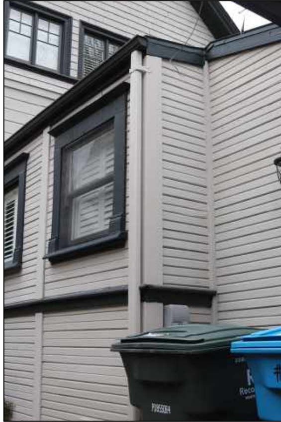
Figure 33: South elevation, southeast corner
