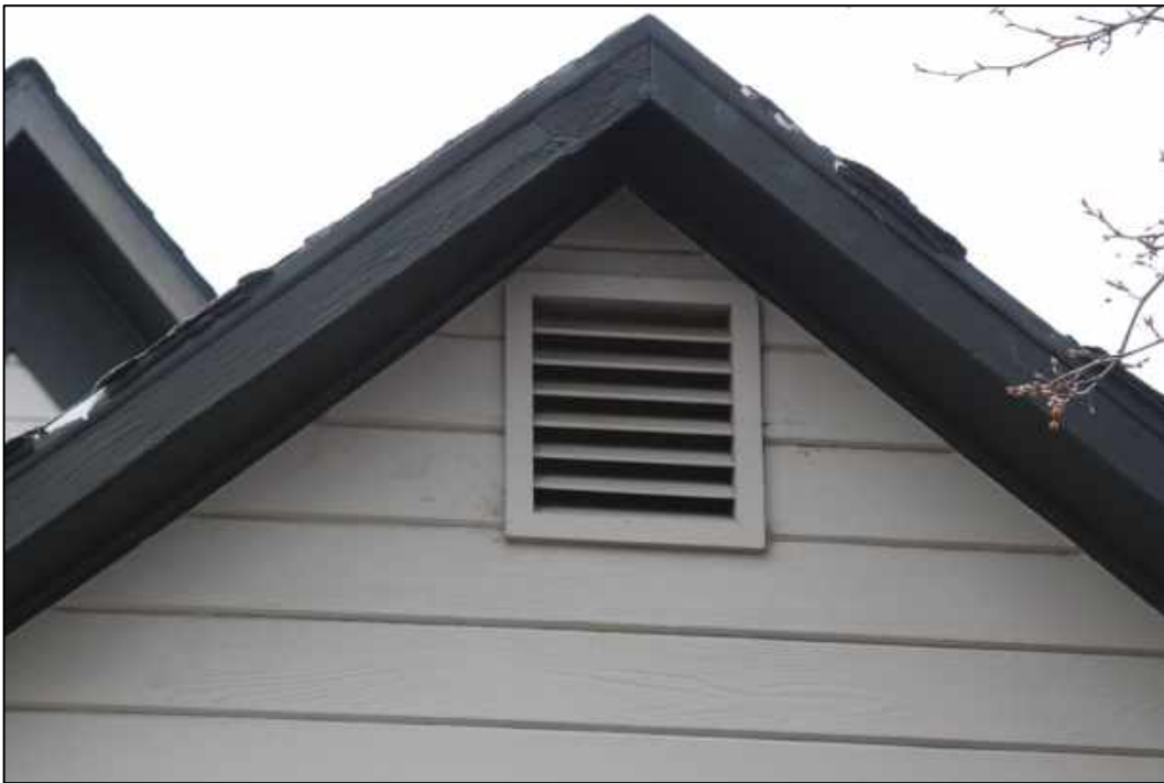
Figure 26: East elevation, vent at gable peak of original section
