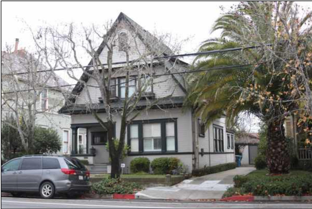
Figure 1: West elevation, fronting B Street (southwest corner)
