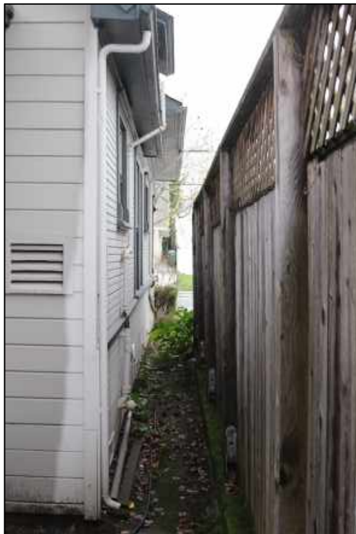
Figure 14: North elevation, property line, looking west
