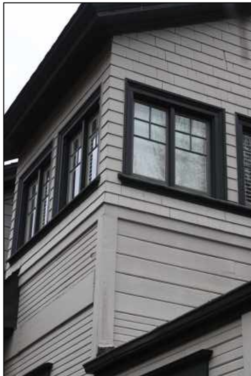
Figure 22: East elevation, upper windows at southeast corner
