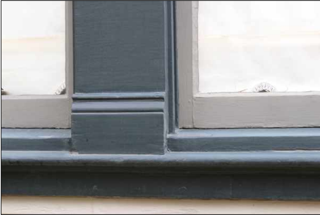
Figure 35: Window trim detail (representative)
