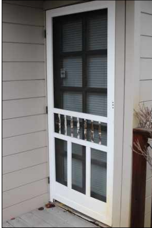
Figure 29: East elevation, back door
