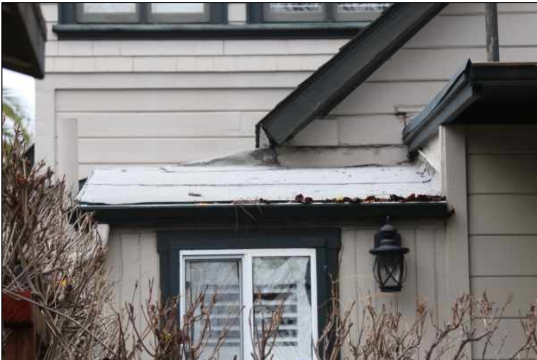
Figure 24: East elevation, infill at corner of original house
