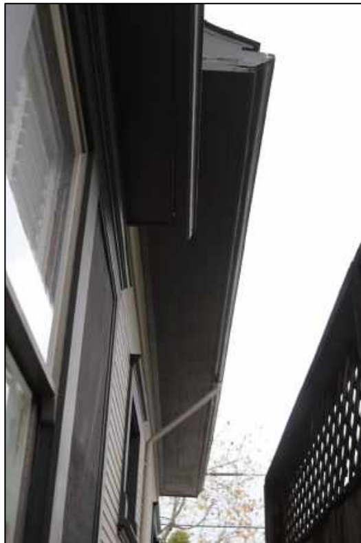
Figure 18: North elevation, eaves
