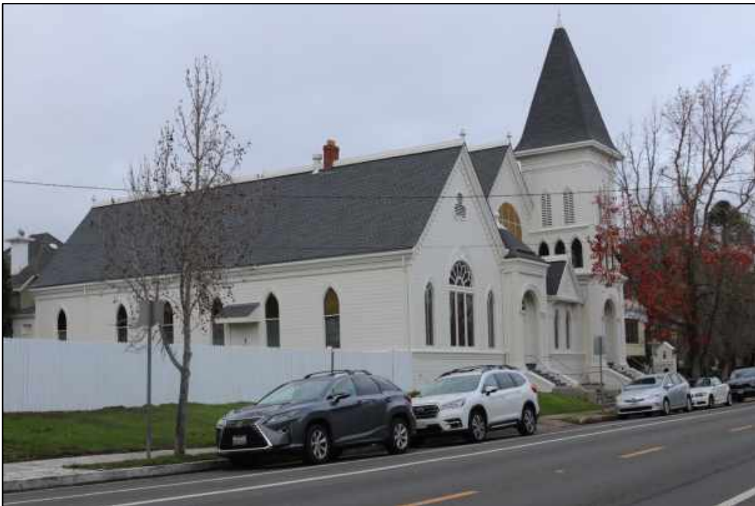
Figure 52: Setting, church to northwest, across B Street
