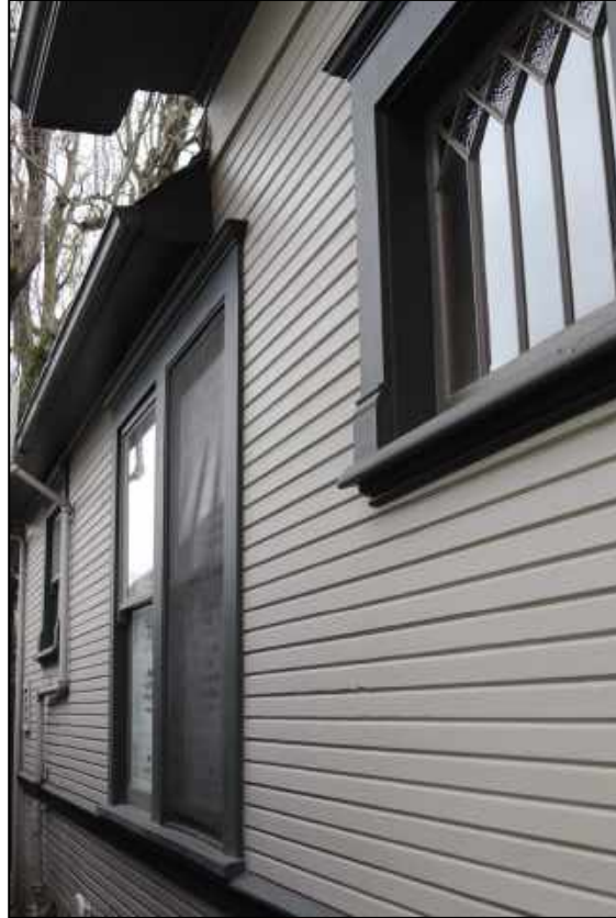
Figure 15: North elevation, windows across junction of addition
