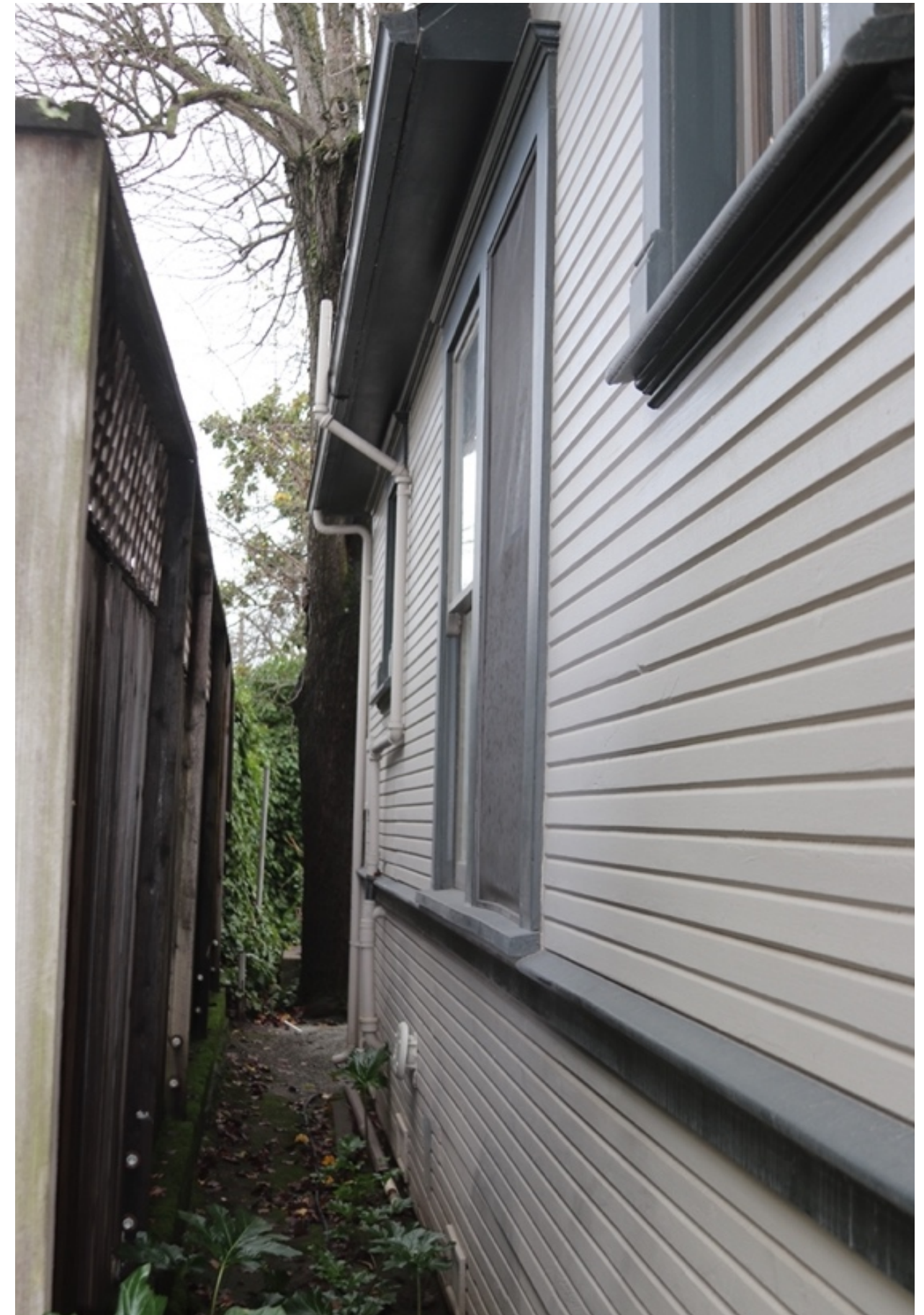
North Elevation looking East
