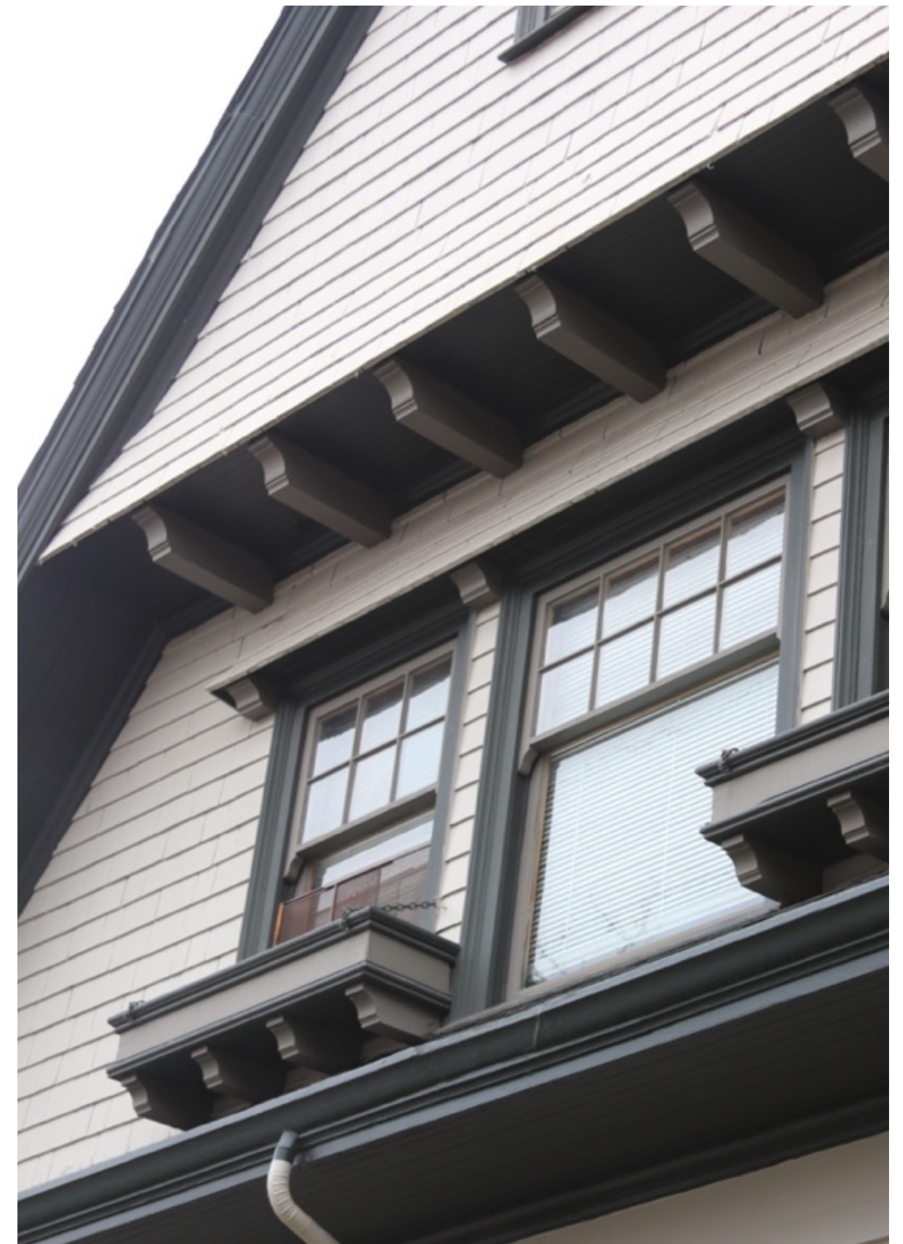
West elevation upper windows
