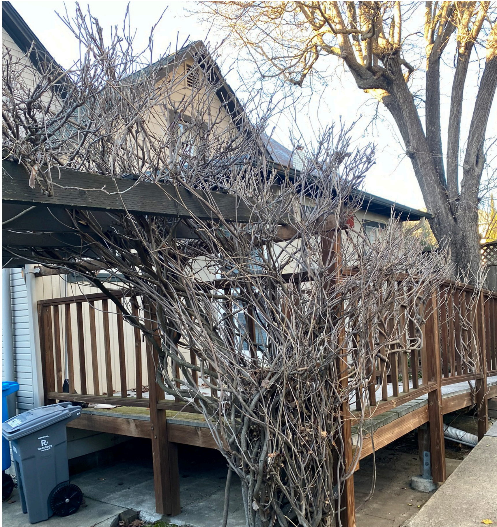
Existing deck and car port
