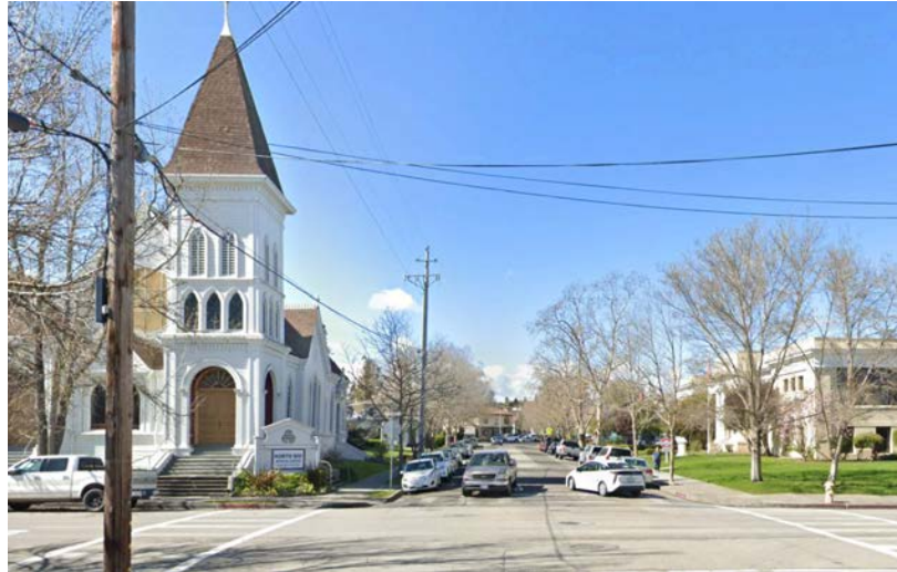
On 5th Street looking northwest (North Bay Revival Center on the left in image)
