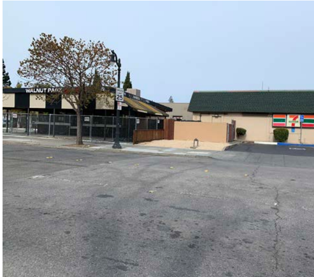
Vacant Structure at Petaluma Boulevard S and D Street
