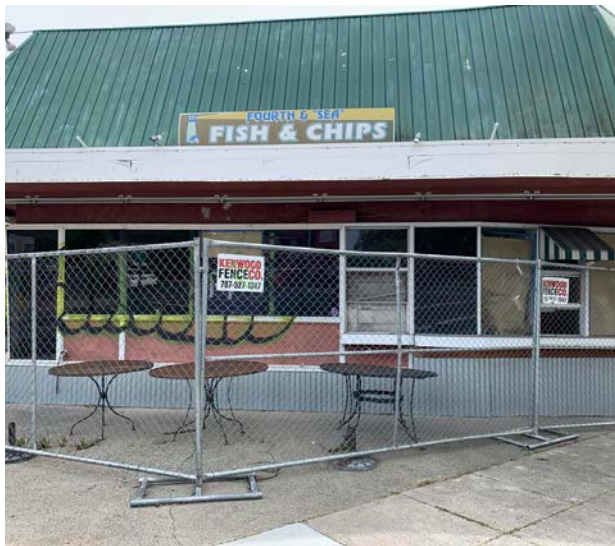
Vacant Structure at 4th Street and C Street
