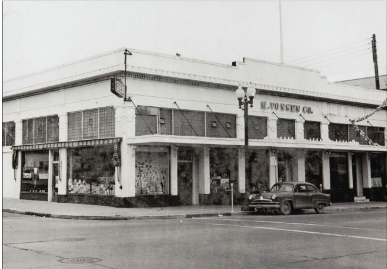
Figure 30: M. Vonsen Co. building by Brainerd Jones, now the City of Petaluma parking garage Source: Sonoma County Library
