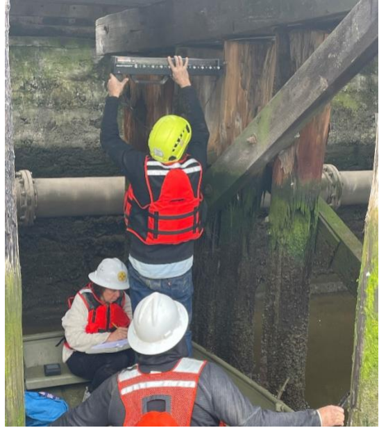
Figure 2. Timber inspectors conduct testing of trestle piles in May 2023.
