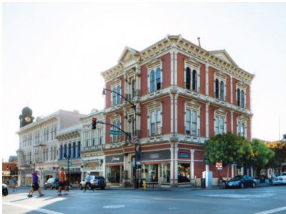
A view looking northeast along Western Ave shows the Mutual Relief Building and Masonic Building
