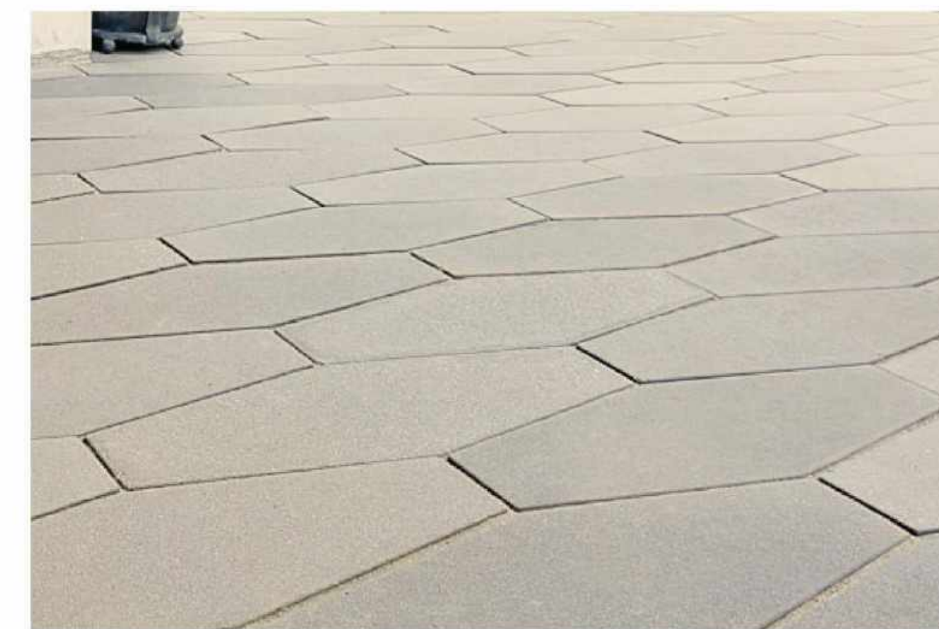
P2 CONCRETE PAVER - TYPE 1 MATERIAL: PRECAST CONCRETE, MORTAR SET SIZE: 24" X 6" X 12" (DIAMOND) COLOR/FINISH: LIGHT BUFF/TAN, SANDBLAST
