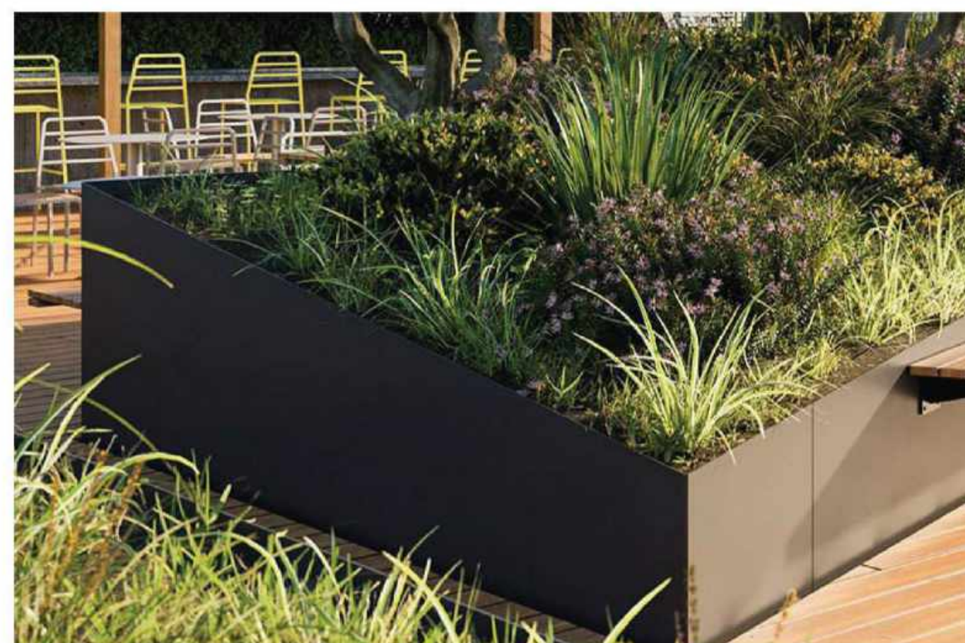
PL3 BUILT-IN PLANTER MATERIAL: METAL SIZE: 36" HT COLOR: POWDERCOAT METALLIC FINISH: STANDARD
