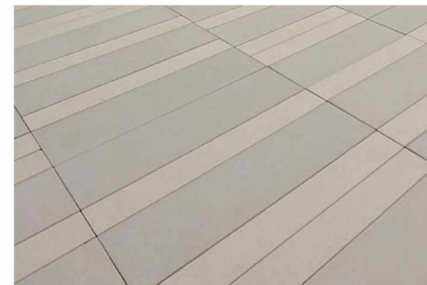
P3 CONCRETE PAVER - TYPE 2 MATERIAL: PRECAST CONCRETE, MORTAR SET SIZE: WIDTHS 6"/12"/24", LENGTHS 48"/60" COLOR/FINISH: LIGHT BUFF/TAN, SANDBLAST
