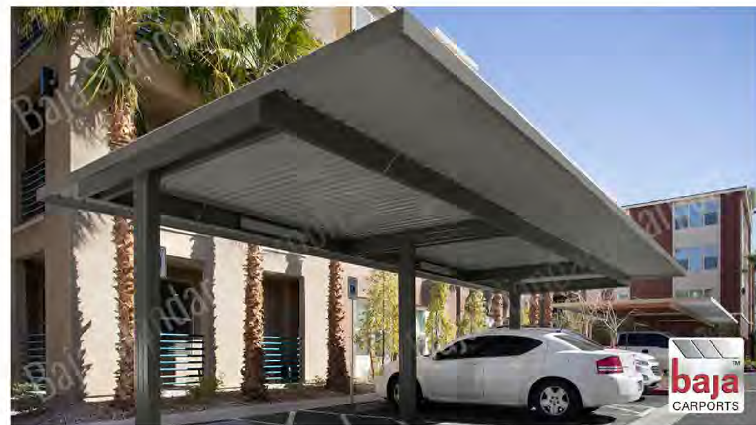
CARPORT EXAMPLE PHOTO PAINT ALL SURFACES TO MATCH ACCENT COLOR (F1) - SEE SHEET A5.1
