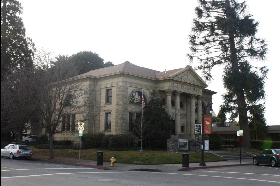
Photo 5: Carnegie Library, looking northwest
