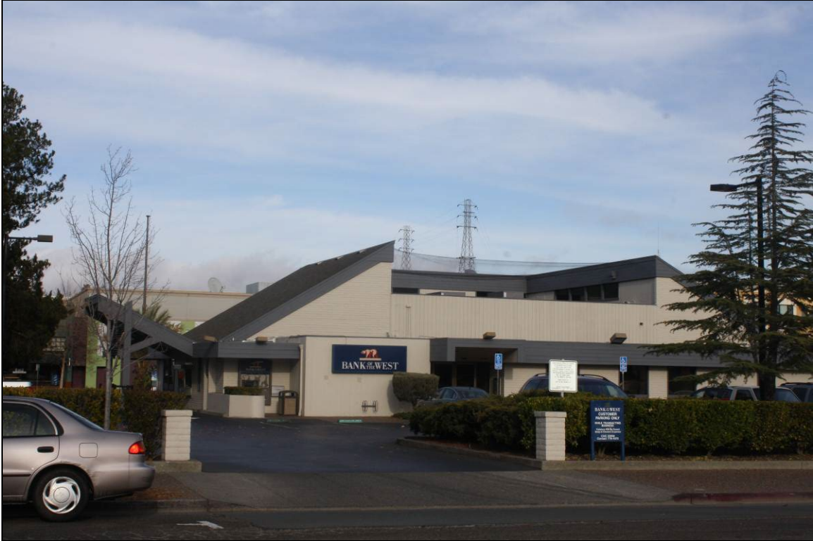
Photo 3: Bank of the West, looking east
