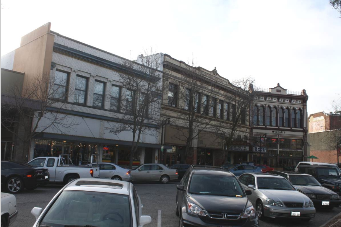
Photo 7: Cast-iron-front buildings, looking northwest
