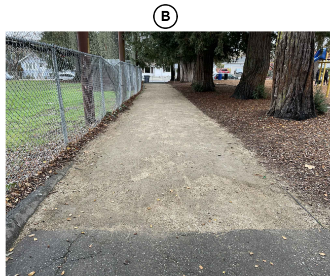
(E) TRANSITION FROM AC TO QUARRY FINES PROTECT QUARRY FINES PATH IN PLACE
