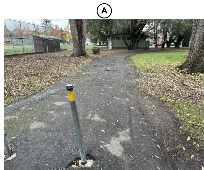
REMOVE EXISTING BOLLARDS
